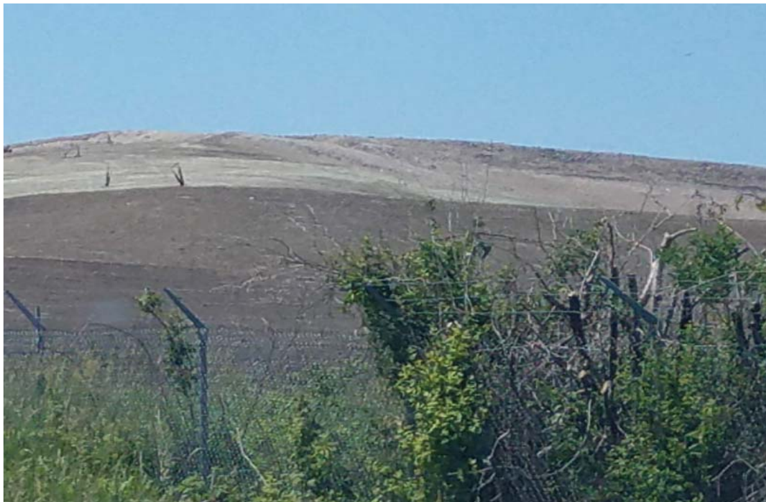
Cap development for Clearwater Pond Expansion
