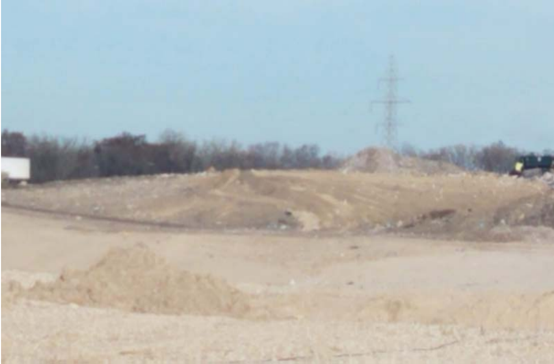
Cover on inactive areas of North Expansion West
