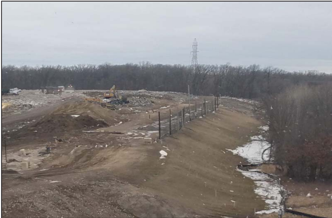
East half of North Expansion Westv (NEW)
