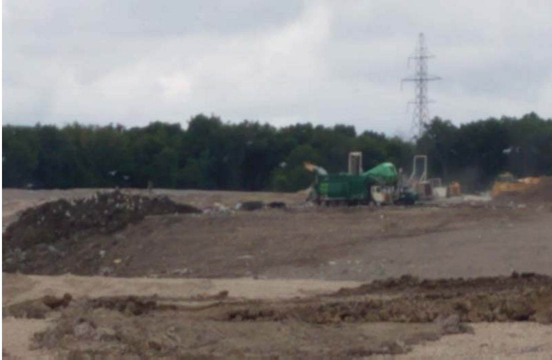
Tipper in center of Phase 1, North Expansion West
