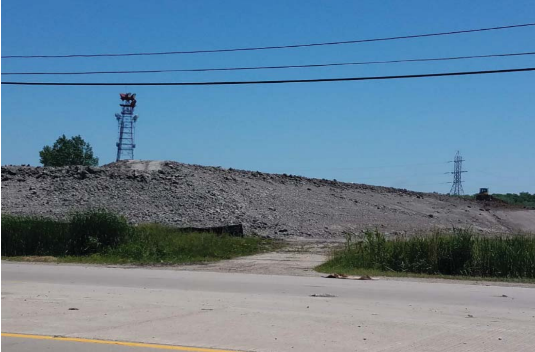
North berm, no control on access to landfill. This has been corrected
