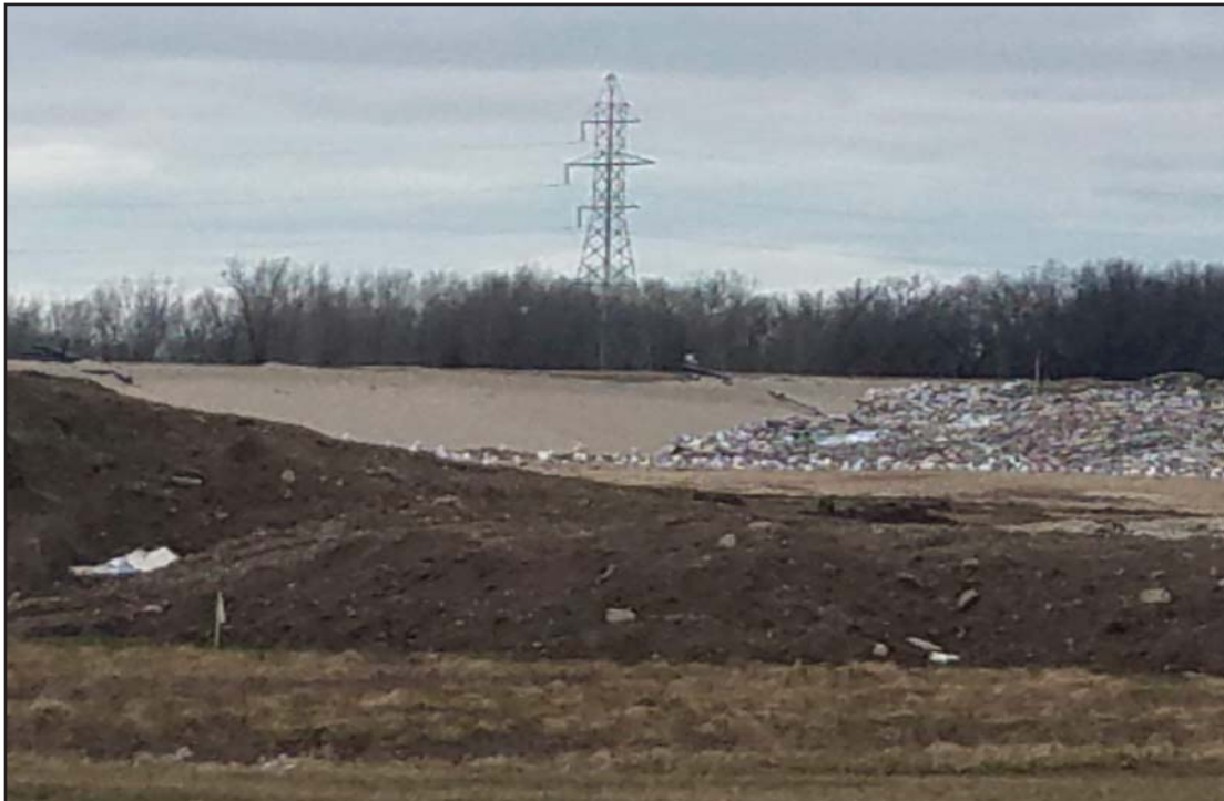
Phase 2 of North Expansion West (NEW) - lyft at North end above fluff layer
