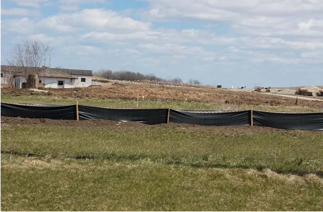
Salvage yard being demolished and contaminated soils being used for daily cover
