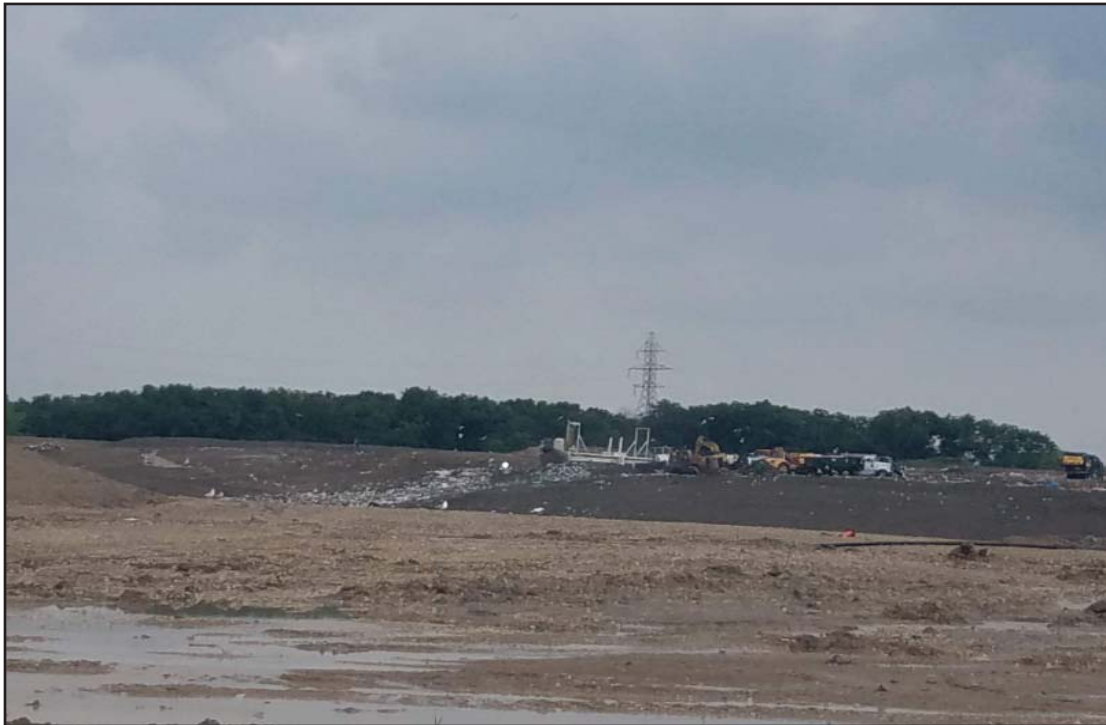
Tipper above working face in North Expansion West (NEW) Phase 2A
