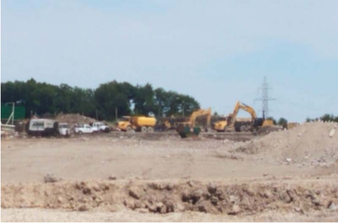
Construction equipment staged outside of Active Area
