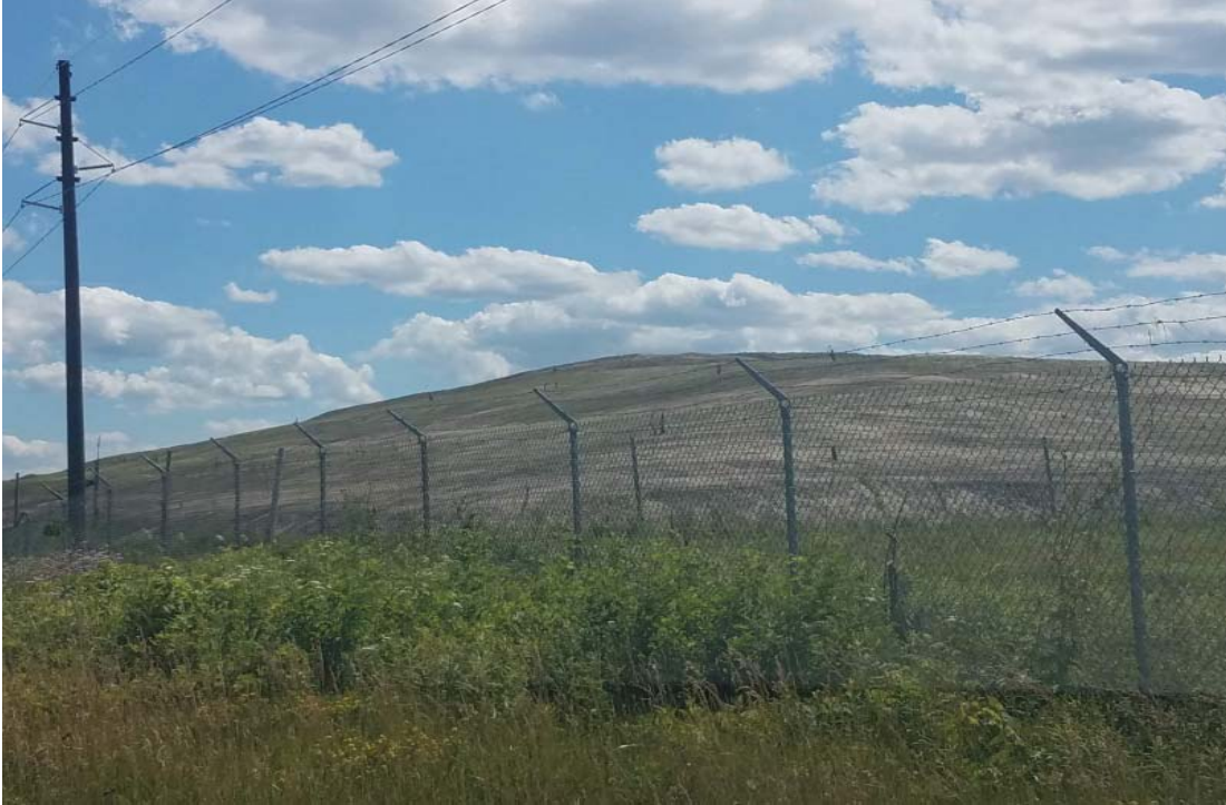
Cap completed on Clearwater Pond Expansion, note vegetation growth
