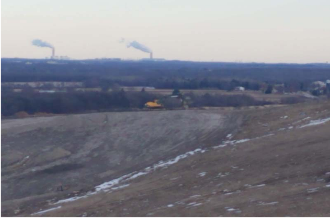
Contractor making connections to gas field in Clearwater Pond Expansion
