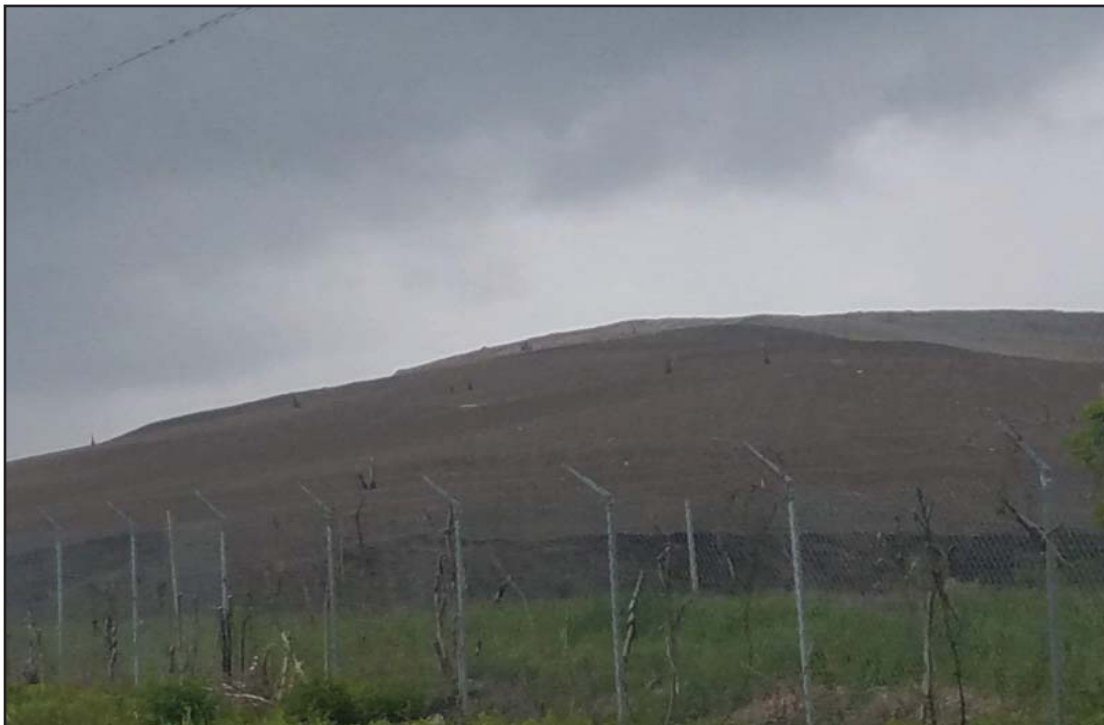
Cap development for Clearwater Pond Expansion
