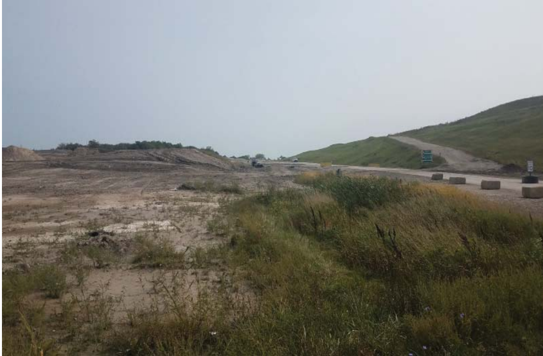
South edge of North Expansion West (NEW)
