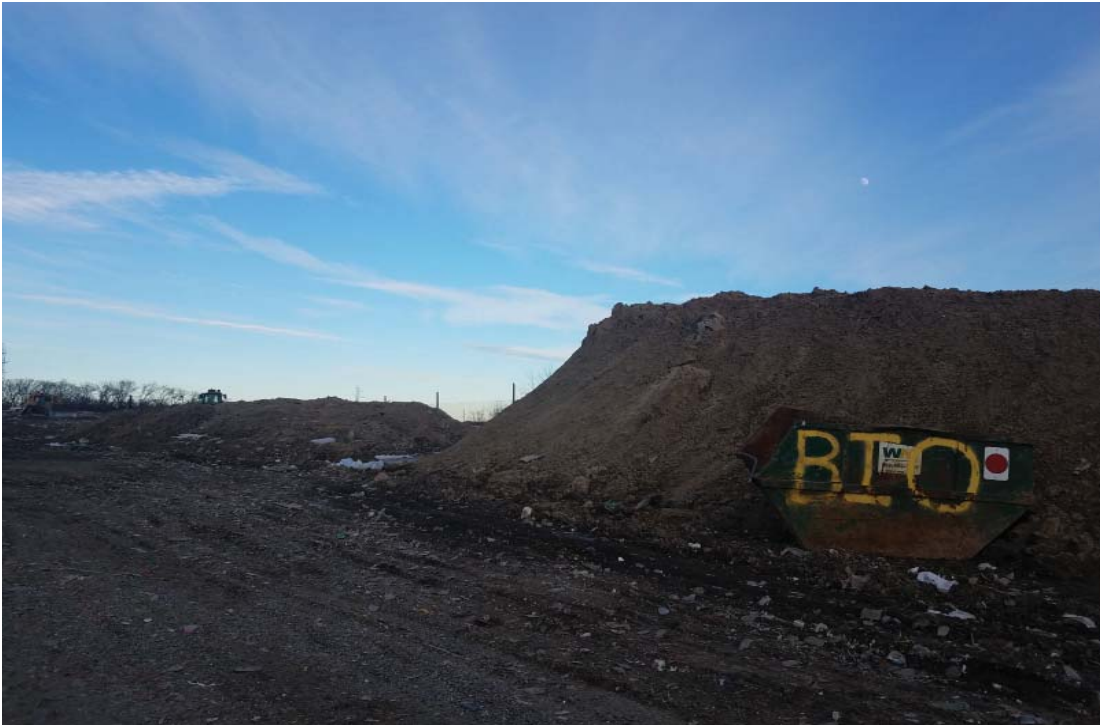
Large BIO soil pile undergoing treatment before use in landfill footprint
