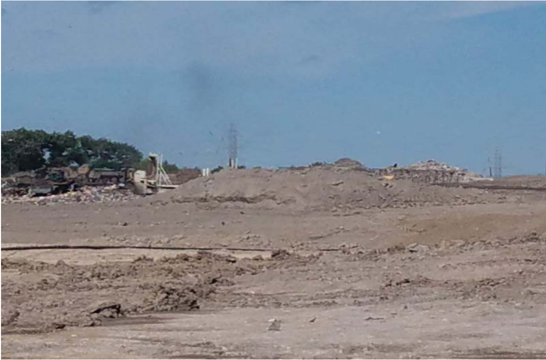
Future phases of North Expansion West prepared for excavation
