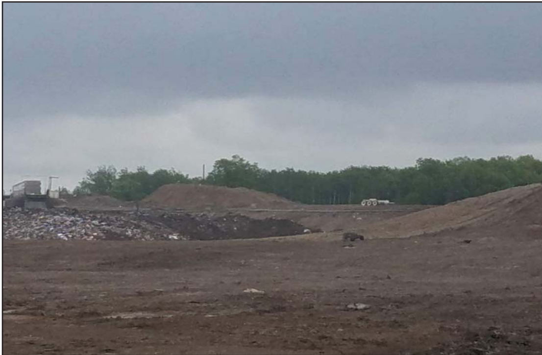
South end of Phase 2 of North Expansion West (NEW)
