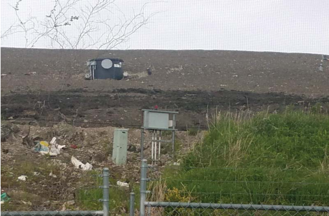
Top soil being applied to Clearwater Pond Expansion East slope
