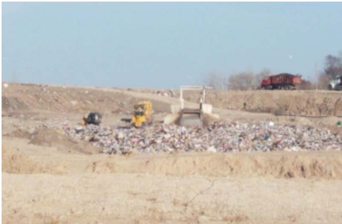
Tipper working in lower area of Phase 2A
