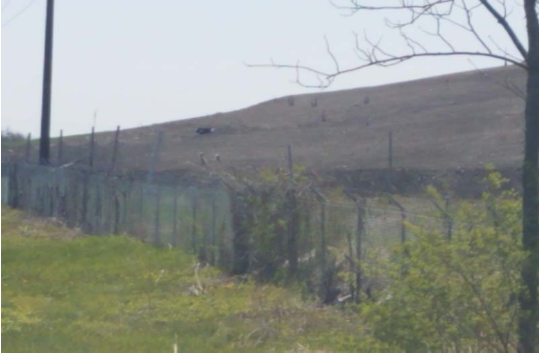
Cap development for Clearwater Pond Expansion
