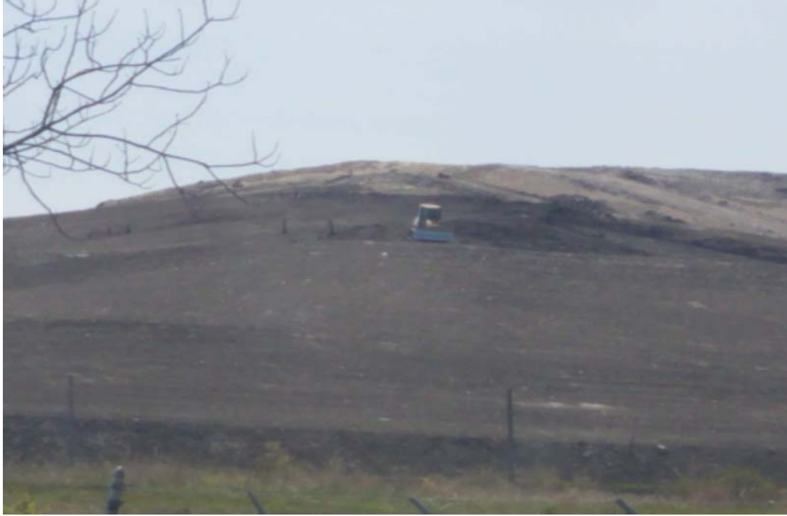
Cap development for Clearwater Pond Expansion
