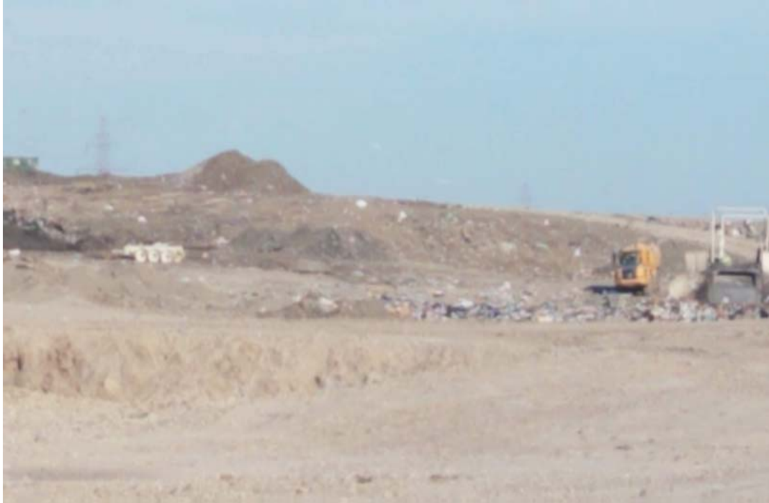
Phase 1B crested above Phase 2A
