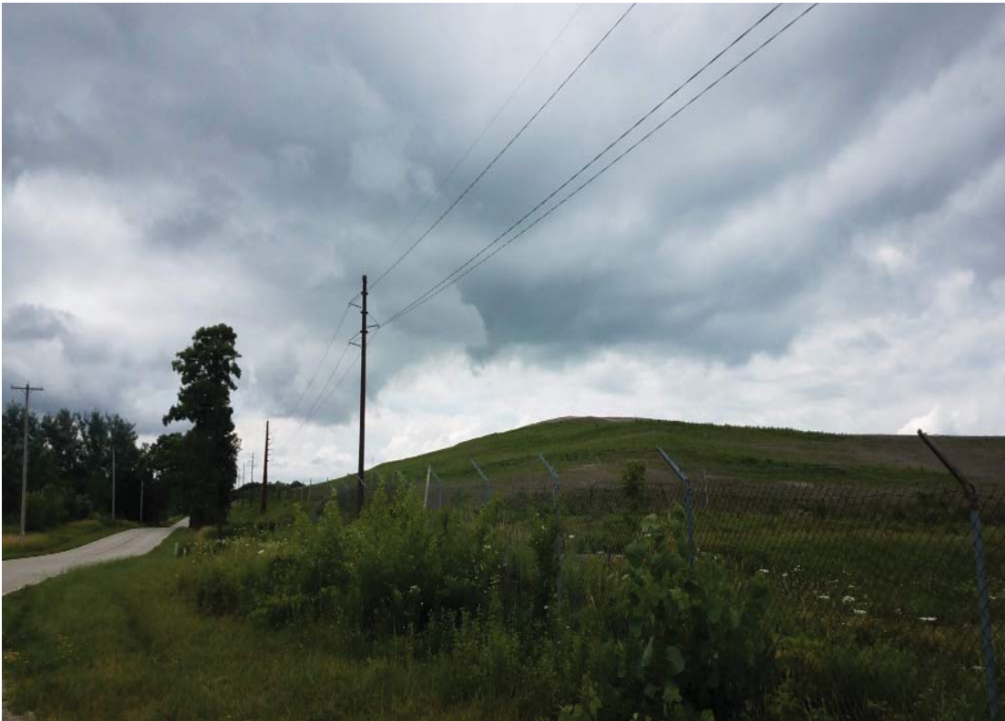
Clearwater Pond Expansion viewed from the North
