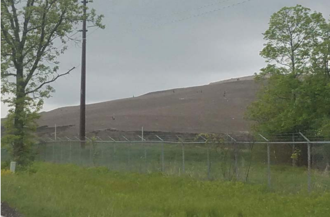
Cap development for Clearwater Pond Expansion
