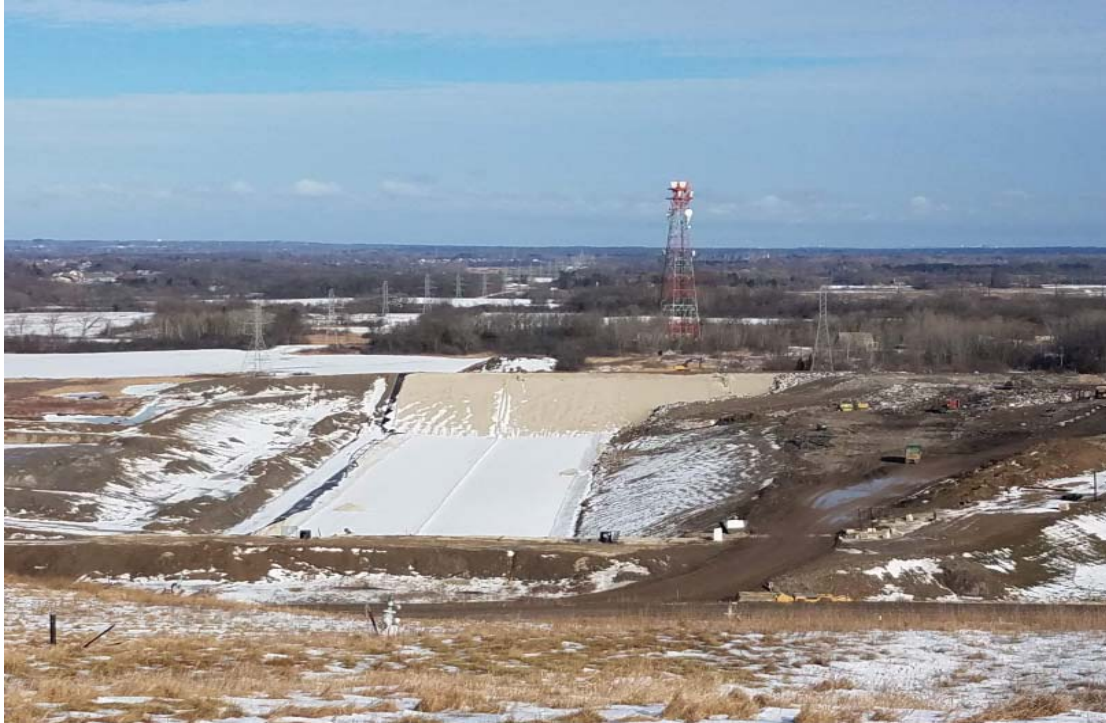
New cell construction completed
