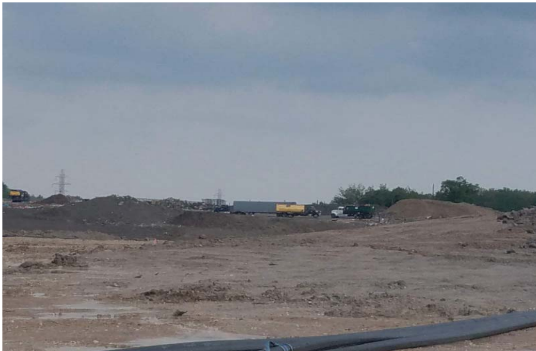
South end of North Expansion West (NEW)
