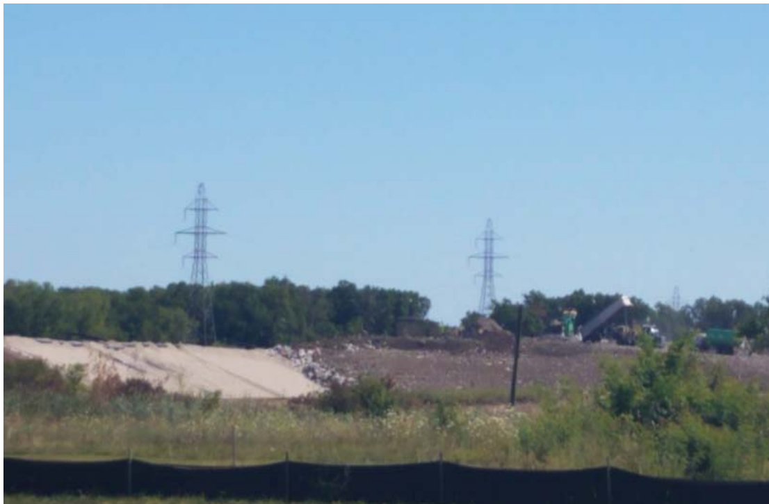
Waste placement moving Westward across Phases of North Expansion West
