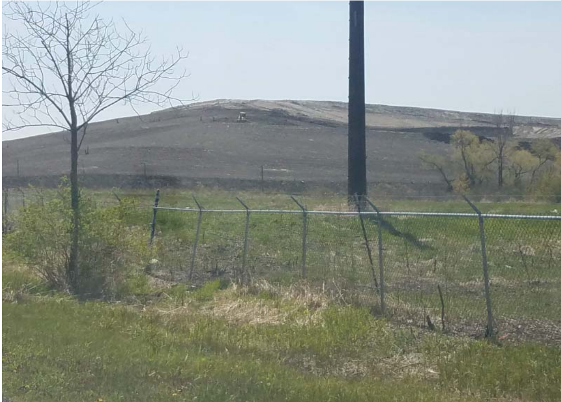
Cap development for Clearwater Pond Expansion
