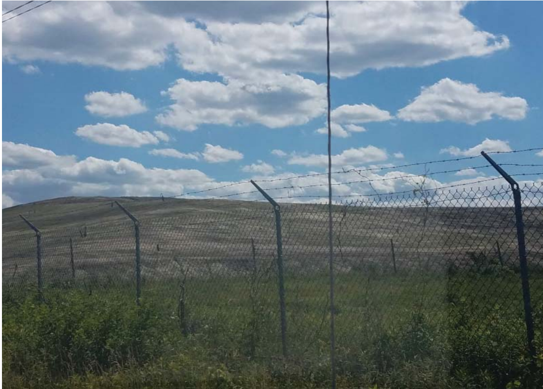
Cap completed on Clearwater Pond Expansion, note vegetation growth
