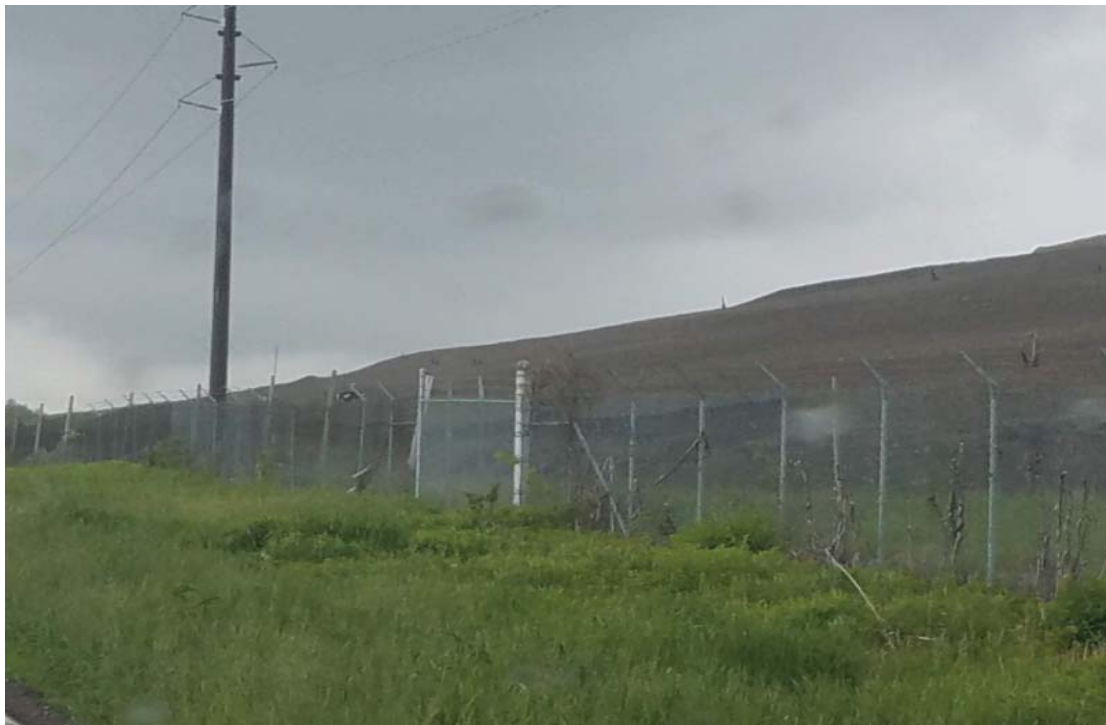
Cap development for Clearwater Pond Expansion
