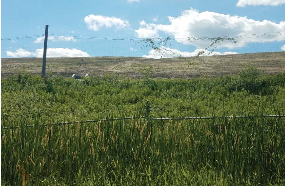
Cap completed on Clearwater Pond Expansion, note vegetation growth
