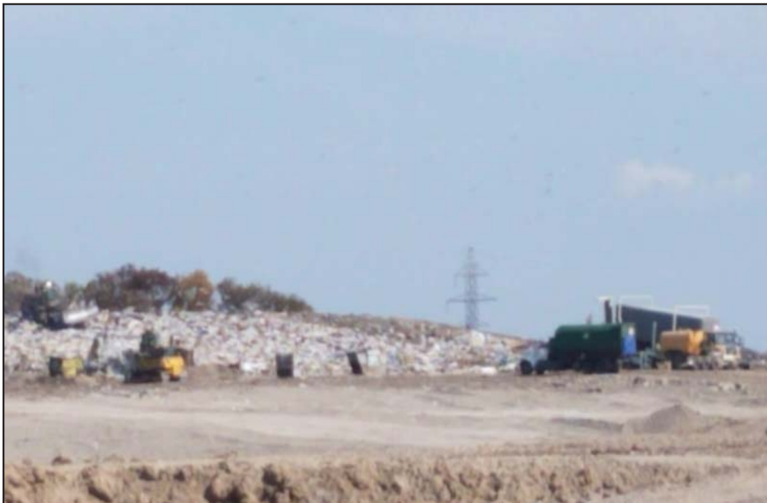
Broad working face in North Expansion West
