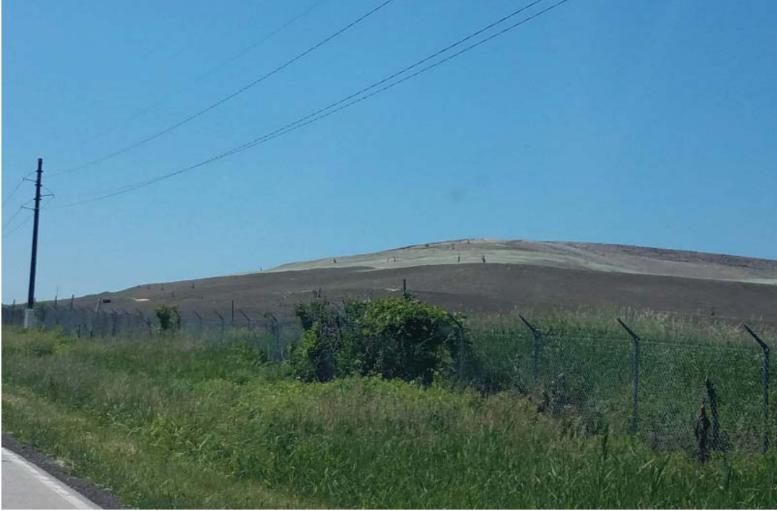
Cap development for Clearwater Pond Expansion
