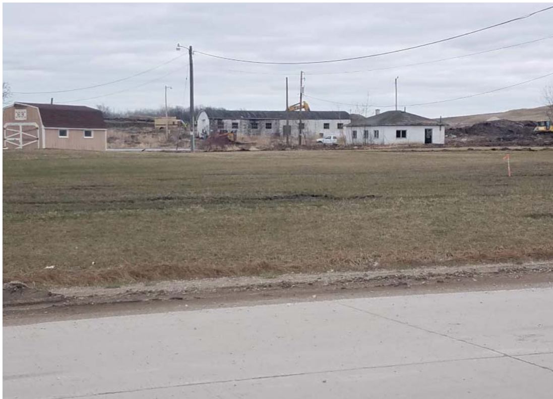
Salvage yard being demolished and contaminated soils being used for daily cover
