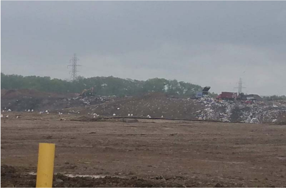
Non-suitable fluff wastes being spread about on Phase 1 of North Expansion West (NEW) prior to cover
