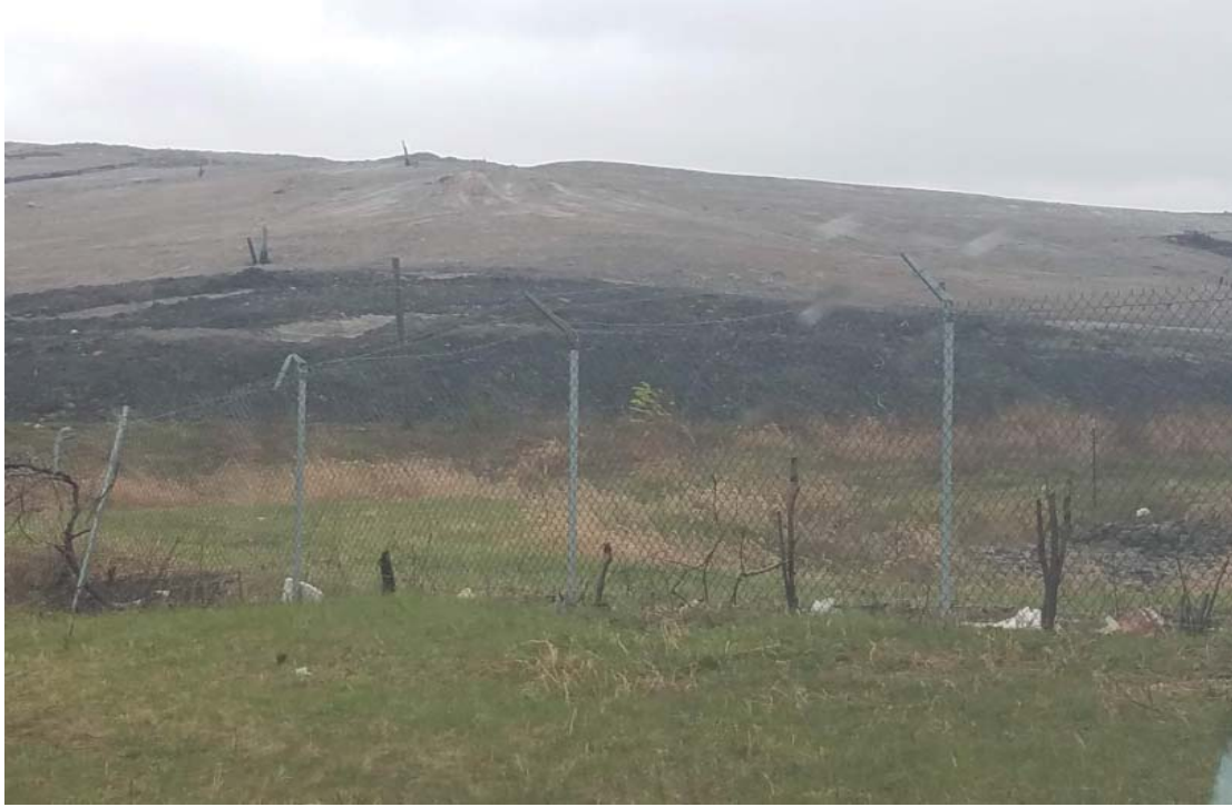
Cap development for Clearwater Pond Expansion
