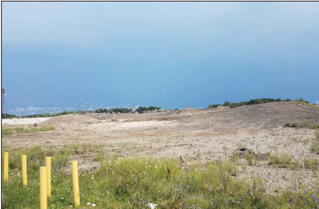
Overview of North Expansion West from West
