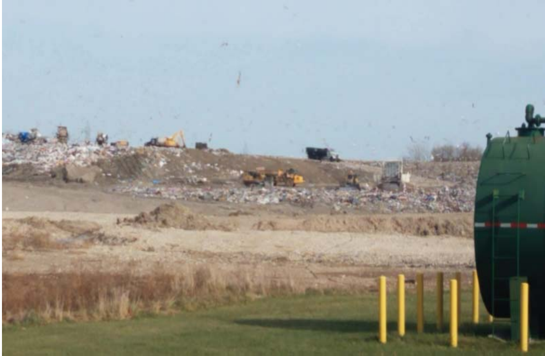
Working face in Phase 2A, with tipper
