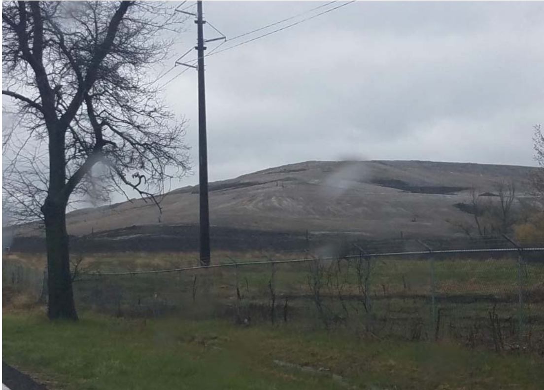
Cap development for Clearwater Pond Expansion
