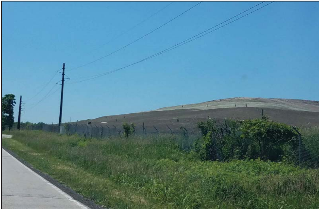
Cap development for Clearwater Pond Expansion
