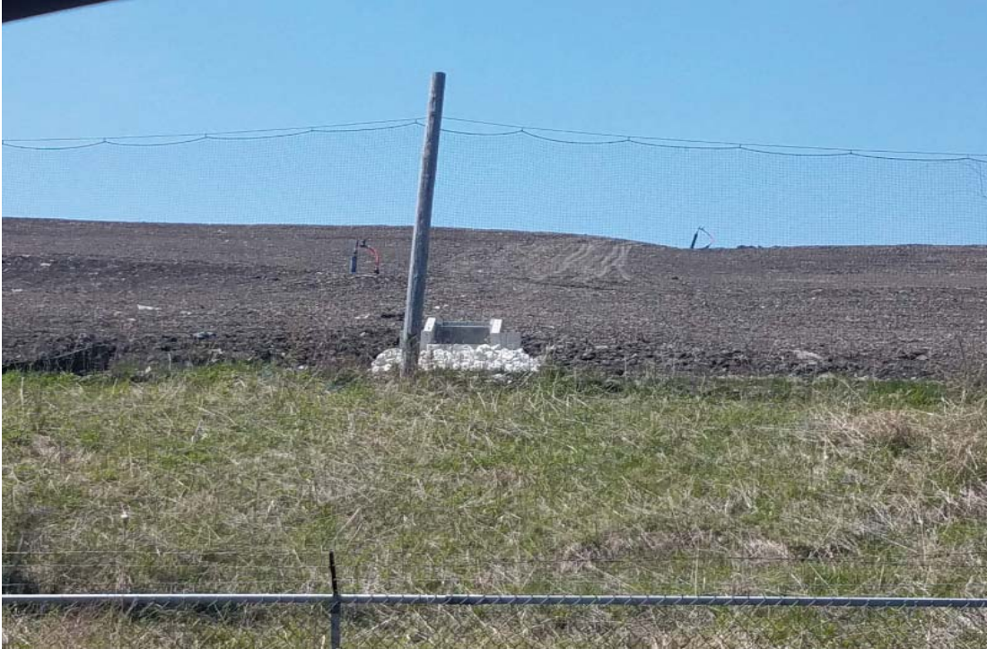
New energy diverter installed in Clearwater Pond Expansion Cap
