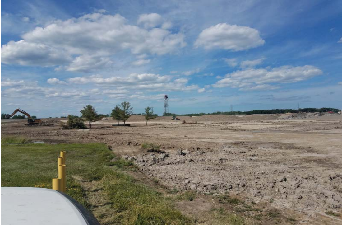
Future excavation of North Expansion West, West of active area
