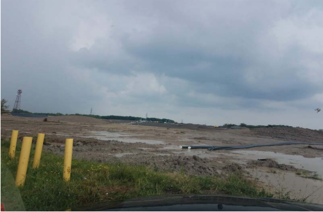
Cleared area of future cell
