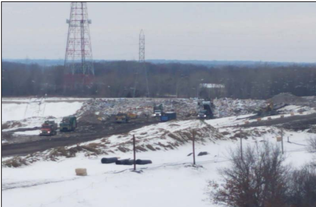
Active area of North Expansion West
