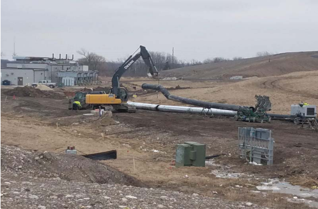
Installation of 24" vacuum line for gas collection in North Expansion West (NEW)
