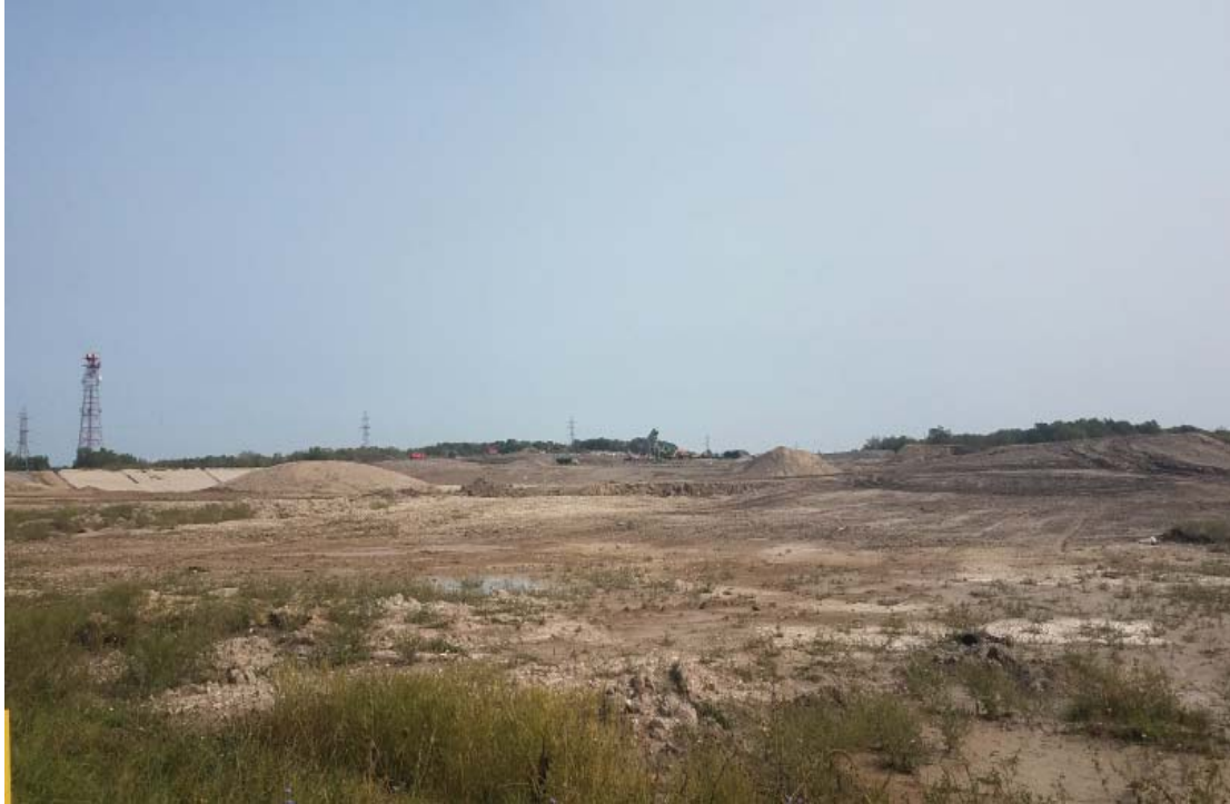
Future Phases of expansion cleared and prepared for excavation
