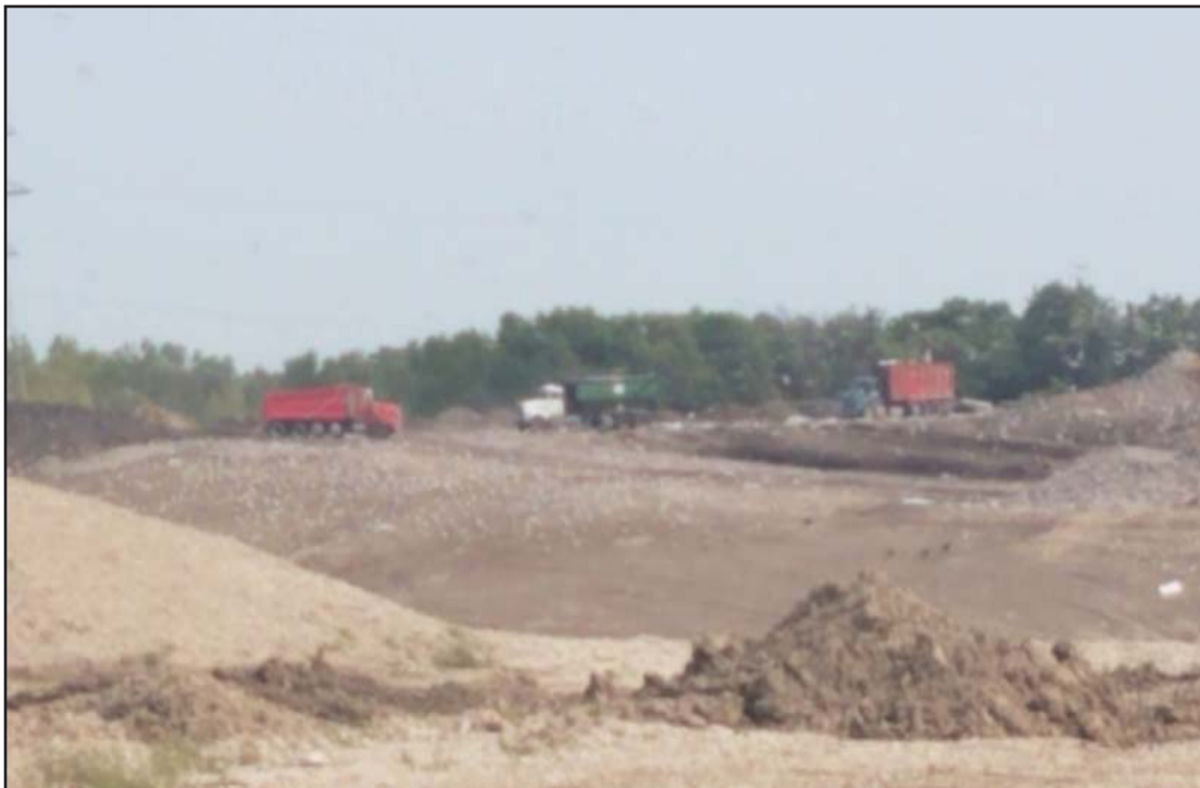
Trucking to North end of Phase 1 of North Expansion West (NEW) for tipping in working face, below grade
