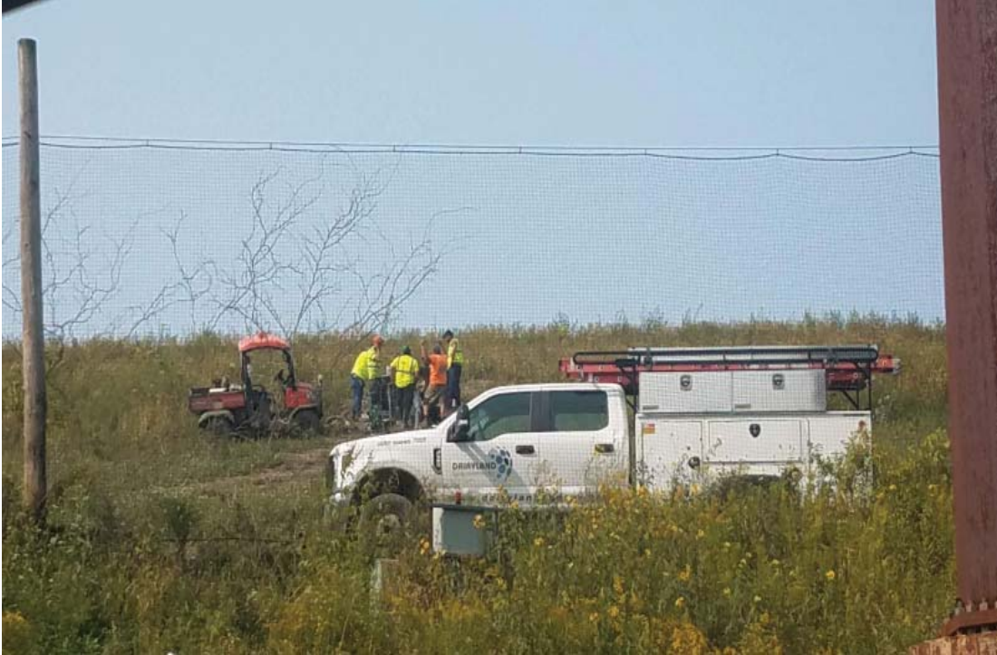
Sideslope riser transducer replacement
