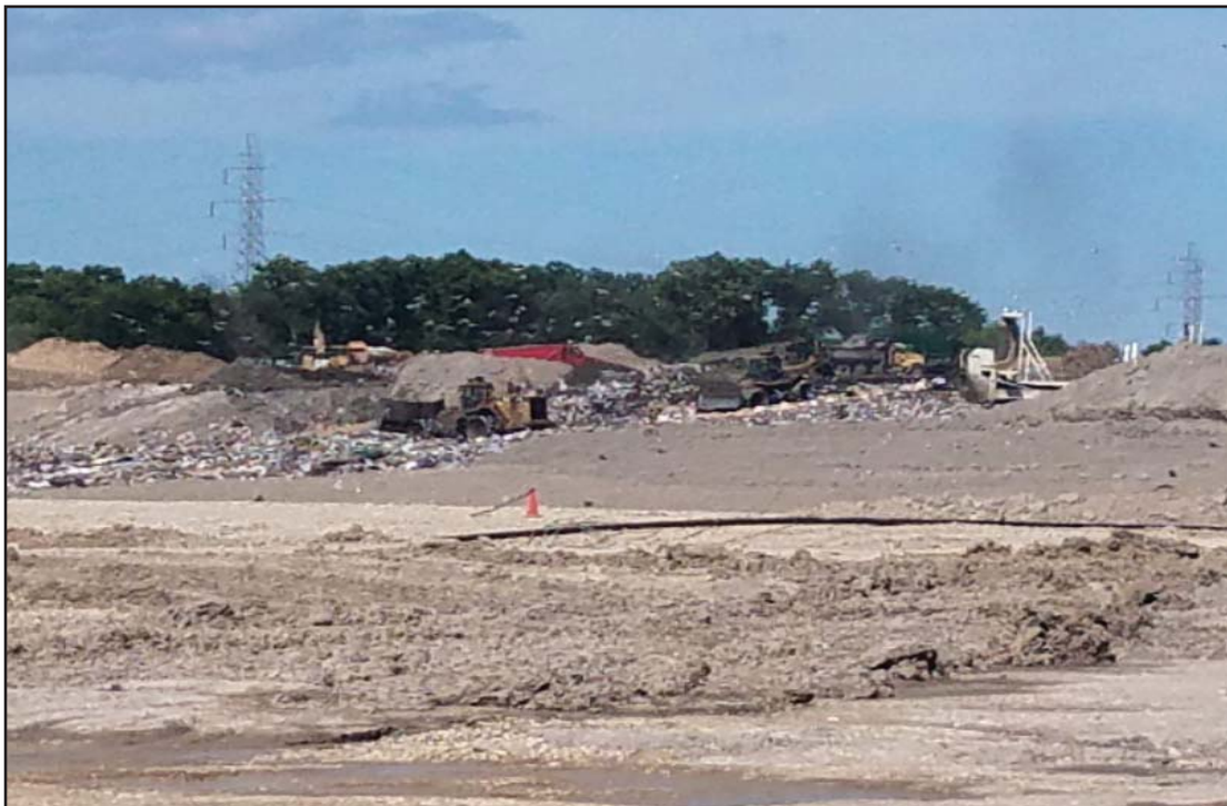
Central view into North Expansion West, working face and tipper in back ground
