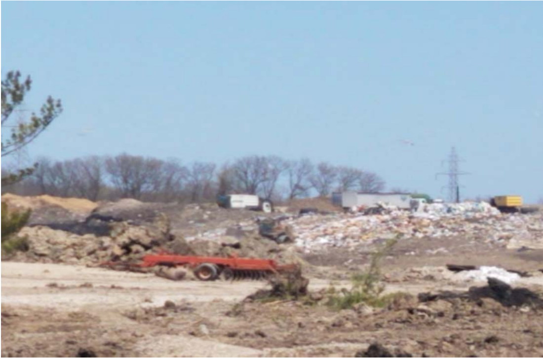
Tipped waste being pushed down into Phase 2
