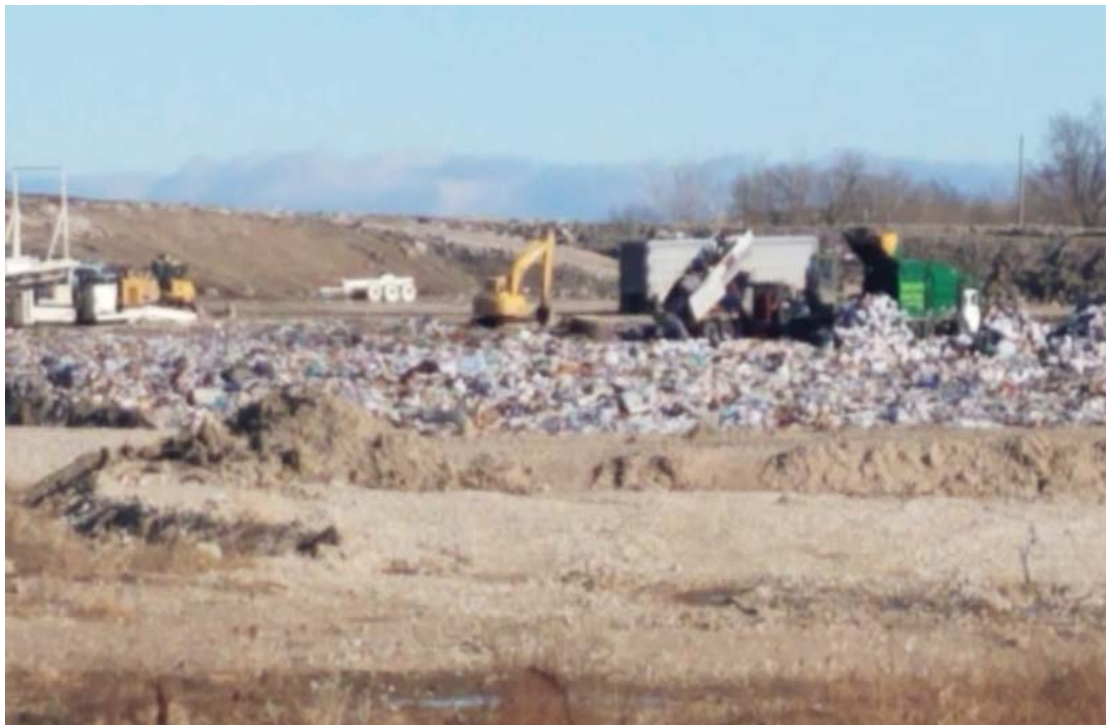
Waste being tipped directly from truck and from trailers on tipper
