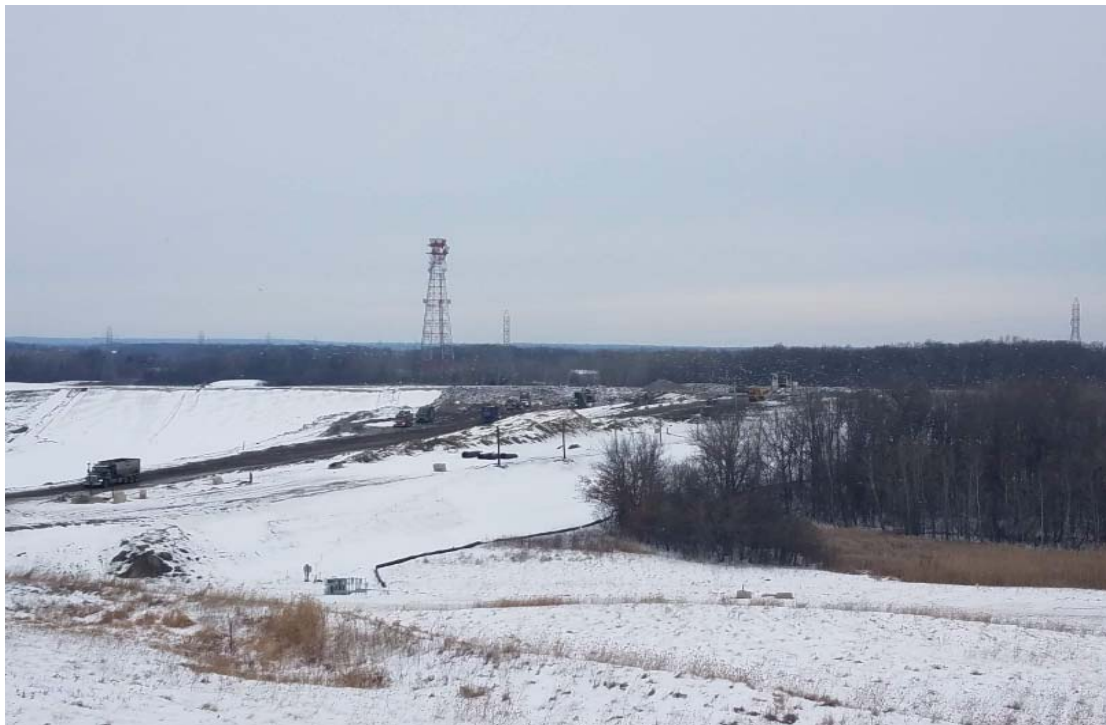
Overview of North Expansion West from the South
