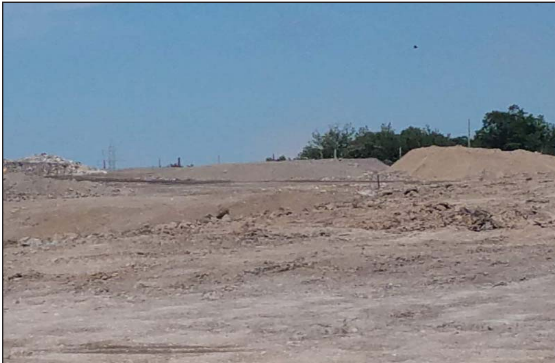
South edge of North Expansion West, prepped for excavation
