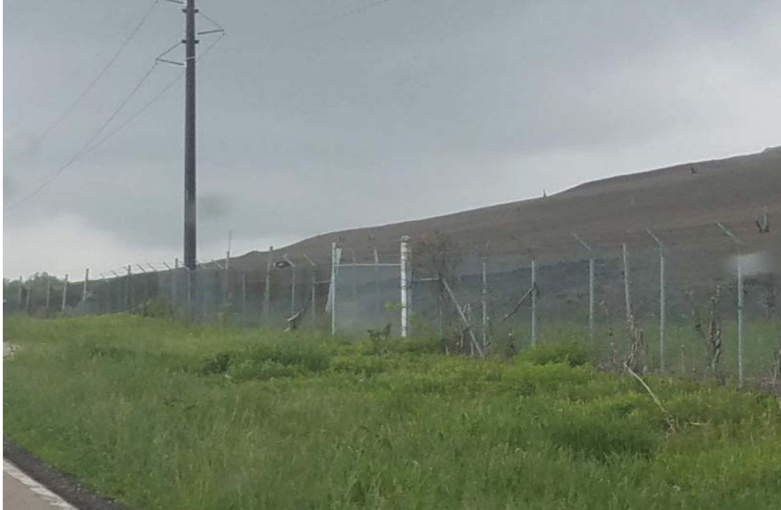
Cap development for Clearwater Pond Expansion
