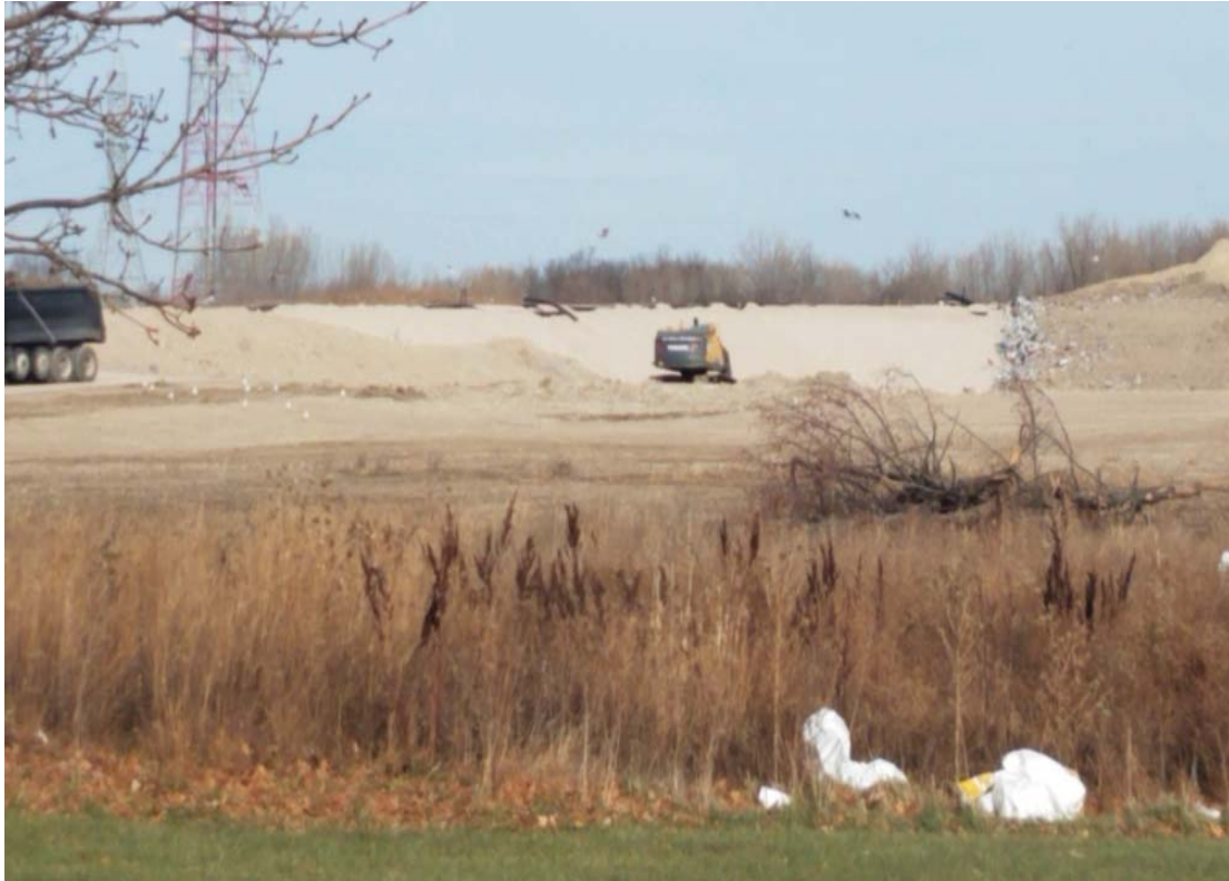
Excavator loading New Berlin Excavation trucks, for off site use by others
