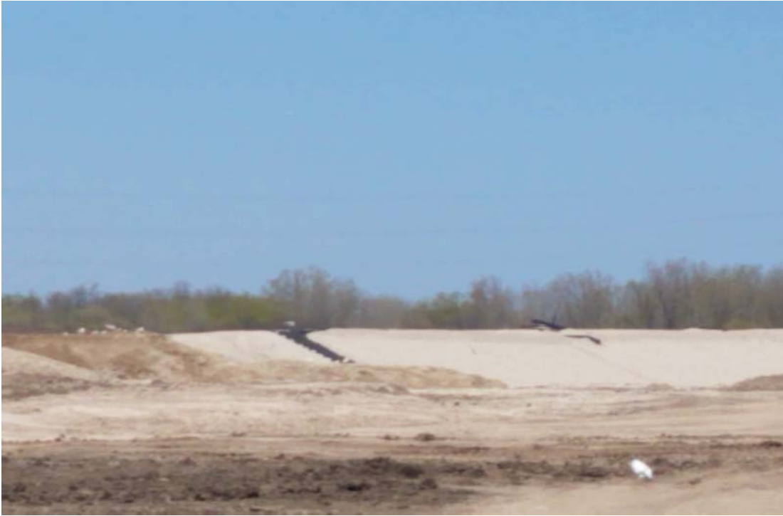
North end of North Expansion West (NEW), no activities
