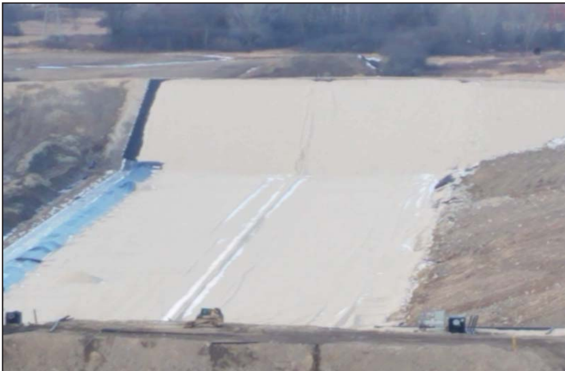
New cell portion of North Expansion West (NEW). Leachate collection system placement on hold while rub sheet placement is relocated
