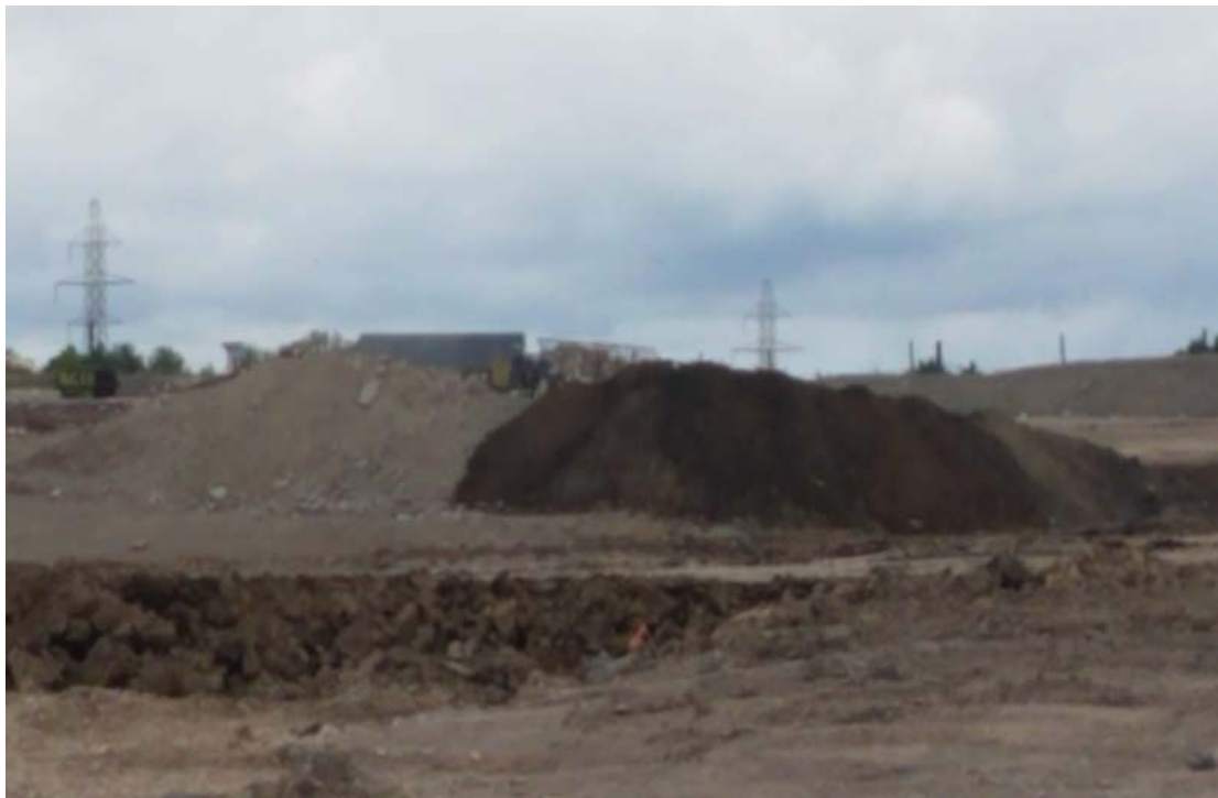
Stockpiled cover in North Expansion West
