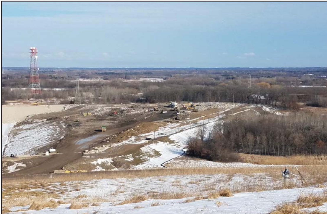
Overview of North Expansion West
