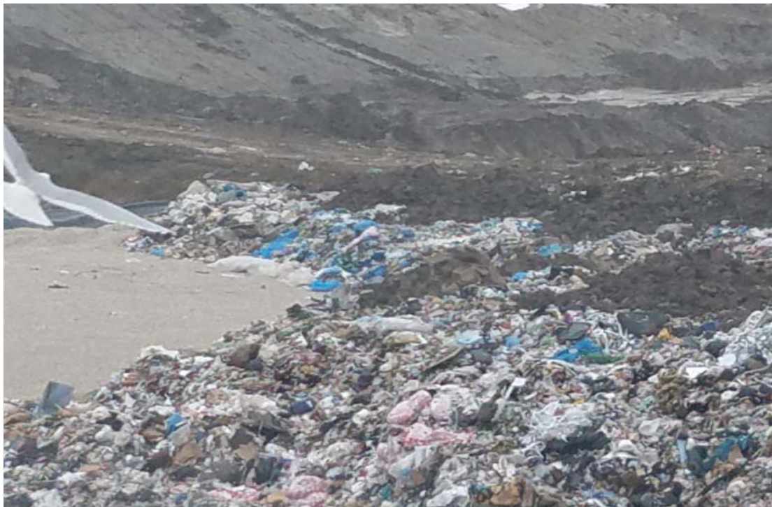
Fluff layer in Phase 2 of North Expansion West (NEW)
