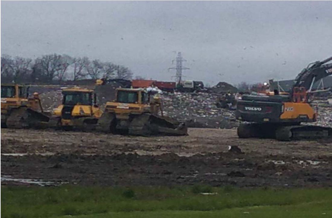
Active area viewed beyond contractor's staged equipment
