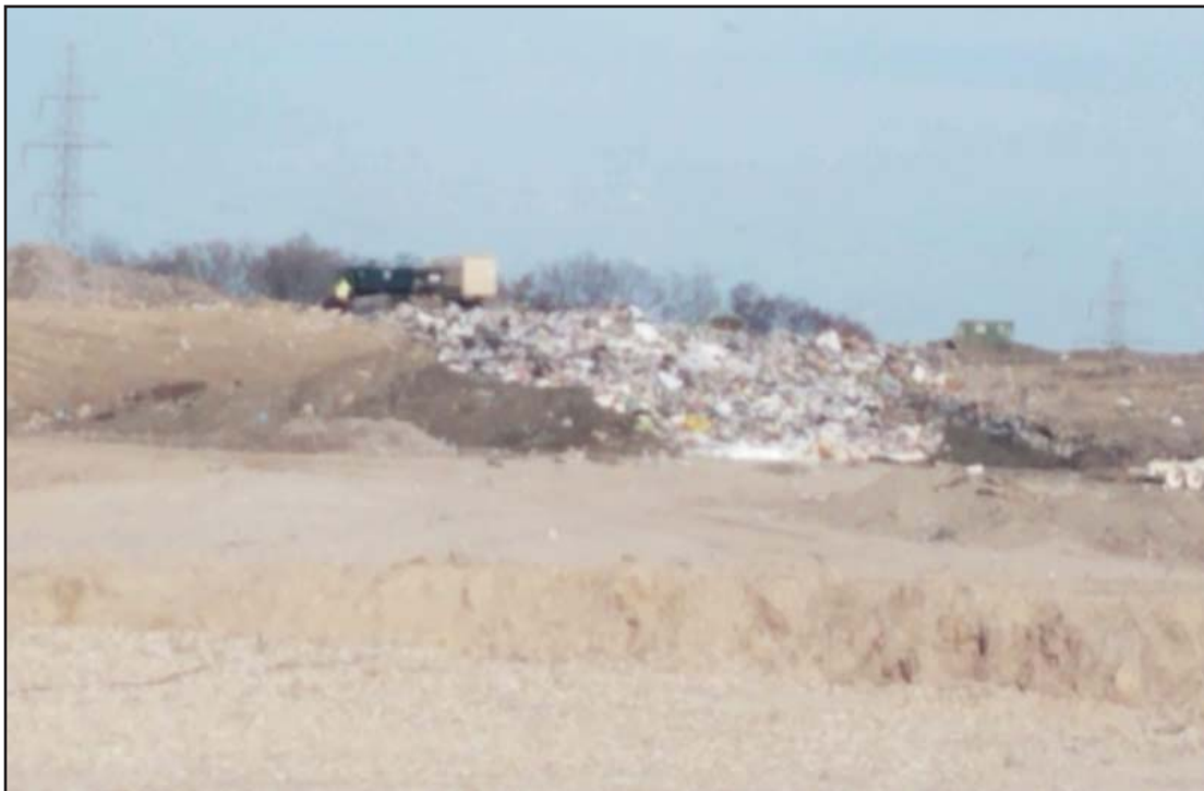
Waste placement in North end of Phase 2A, above grade
