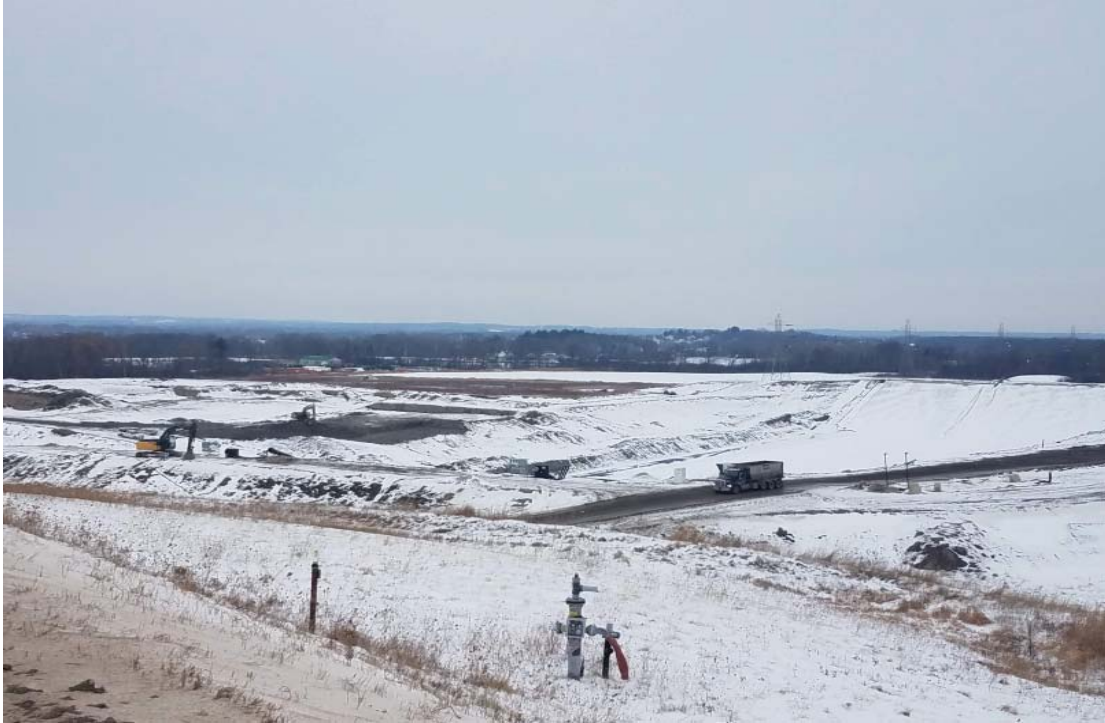
Clearwater Pond Expansion viewed from the West
