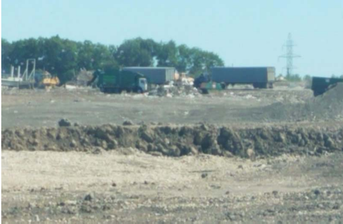
Truck traffic across North Expansion West
