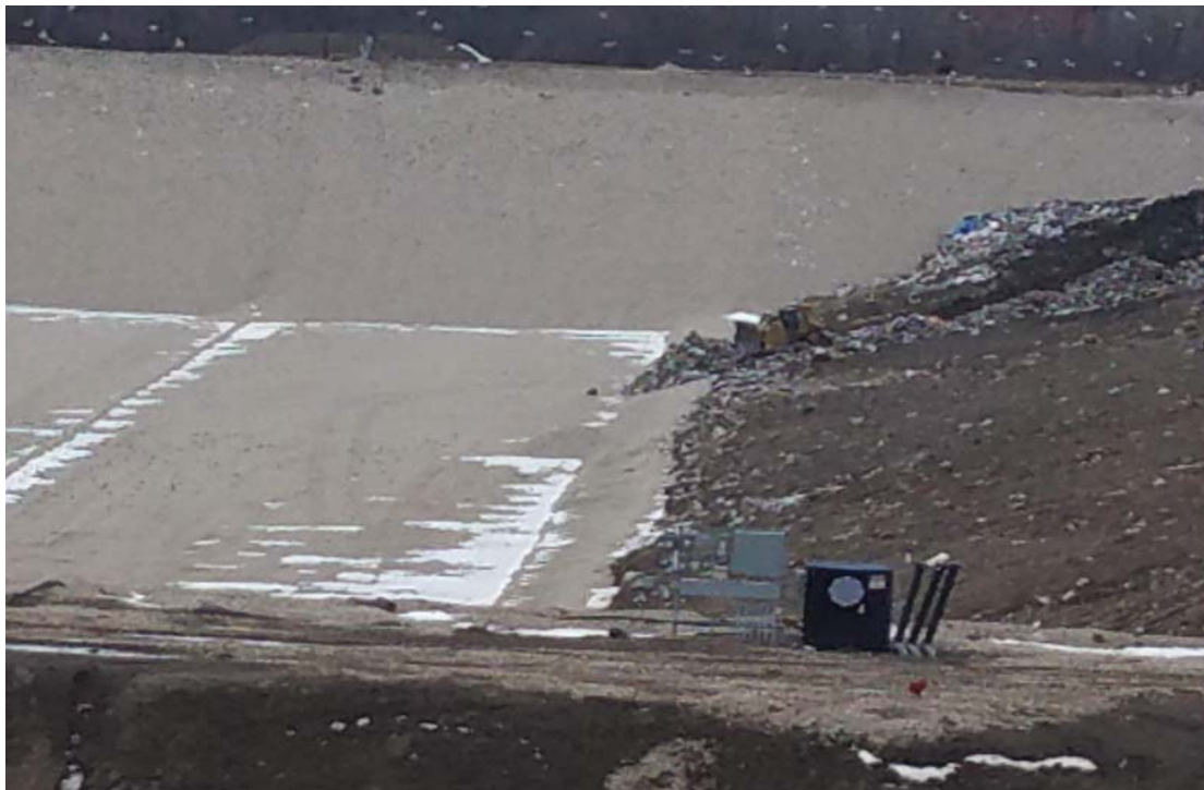
Phase 2 A of North Expansion West(NEW) receiving first tipping/push of fluff layer
