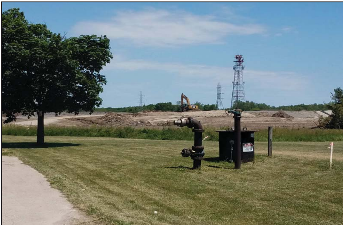
Berm construction ongoing
