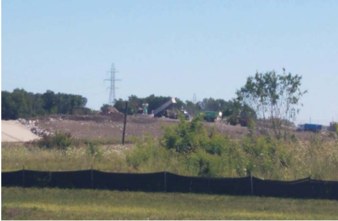
Working face viewed from US 45
