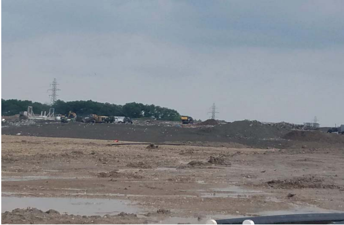
Active are in center of North Expansion West (NEW)
