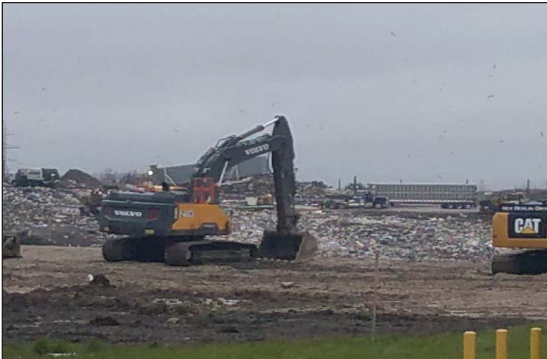
North Expansion West (NEW) viewed from gas plant
