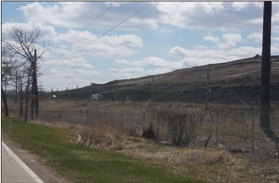
Restoration of Clearwater Pond Cap
