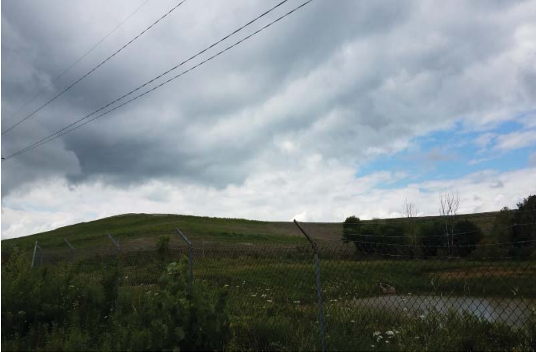
Clearwater Pond Expansion viewed from the North
