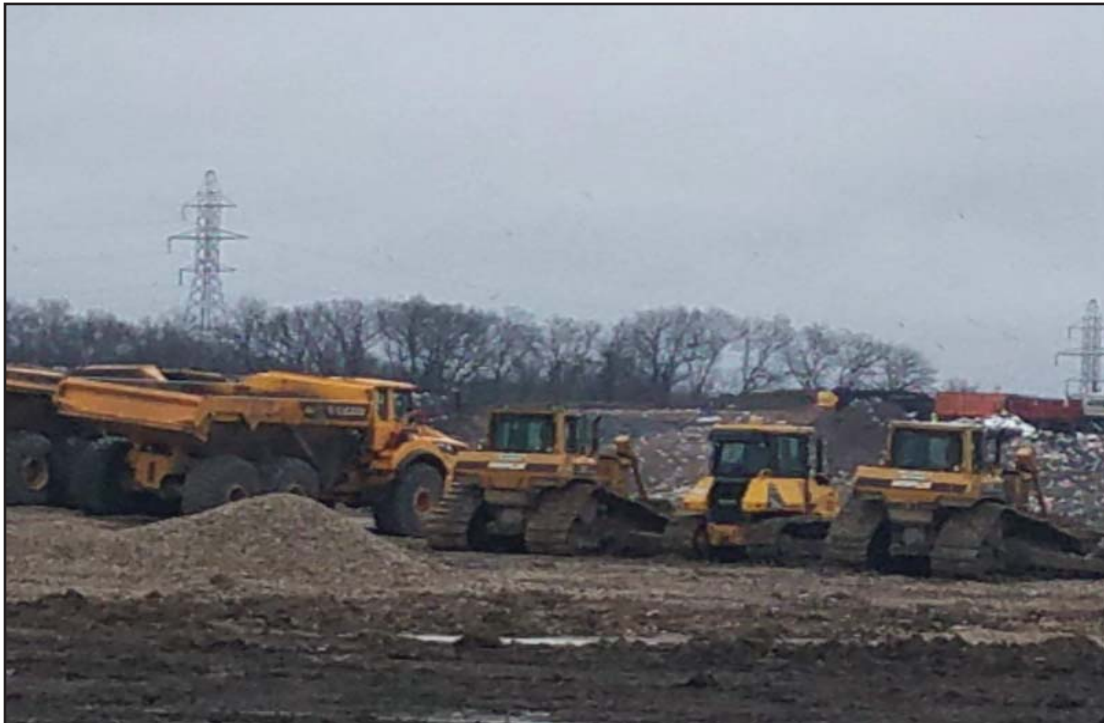
Staged equipment of contractor
