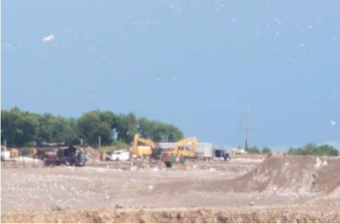
Contractor equipment staged out of the way
