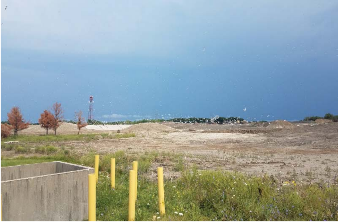
Overview of North Expansion West from South
