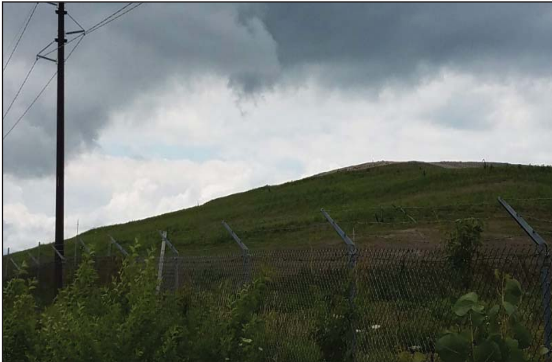
East slope of Clearwater Pond Cap
