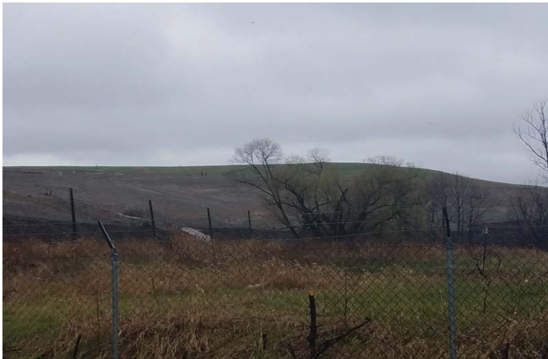
Cap development for Clearwater Pond Expansion
