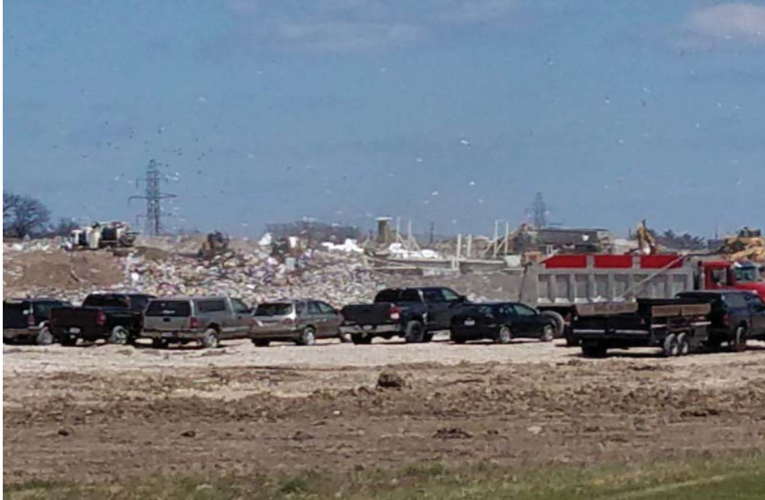
North Expansion West (NEW) viewed from gas plant
