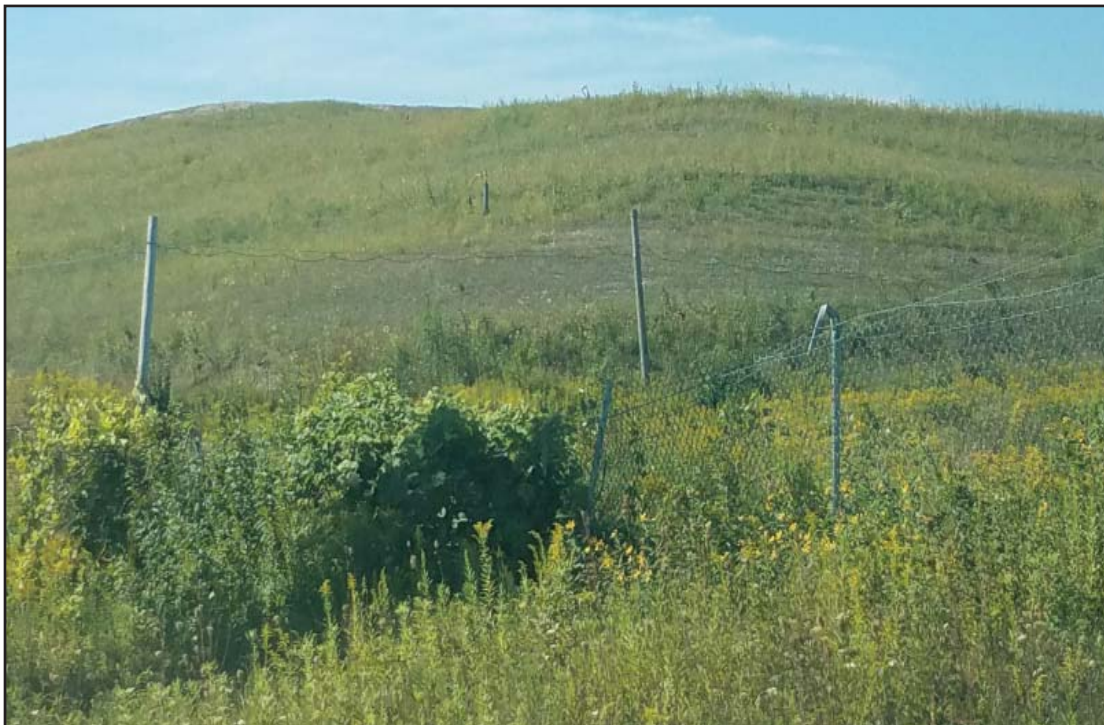
Northeast corner of Clearwater Pond Expansion, vegetative growth good except for tip of the corner
