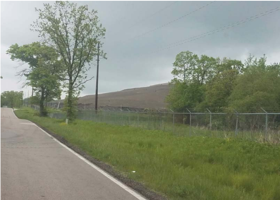
Cap development for Clearwater Pond Expansion
