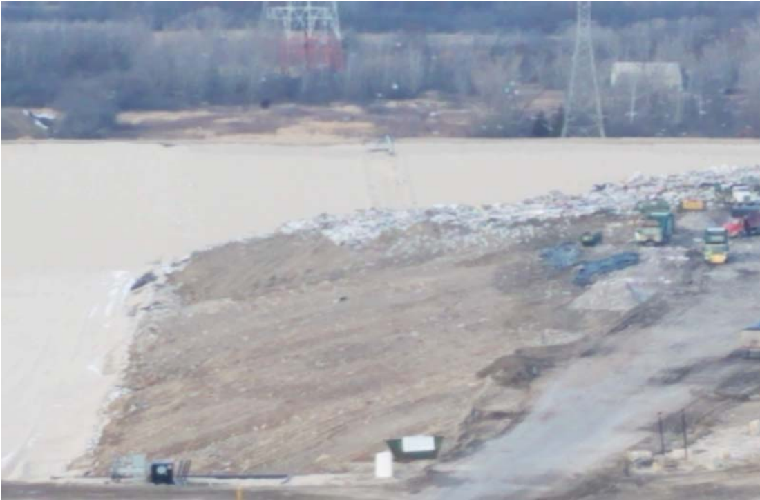
West slope of North Expansion West above new cell
