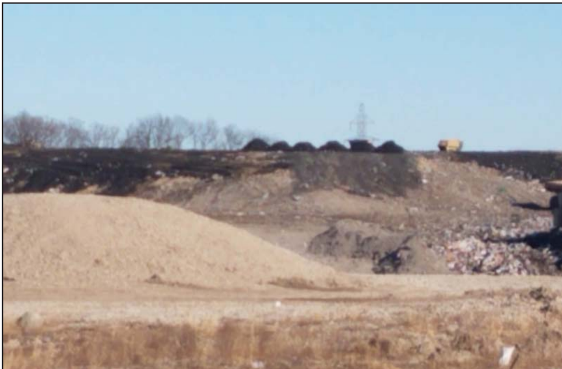
Previous Working face in Phase 1B, covered with dredging material from off site
