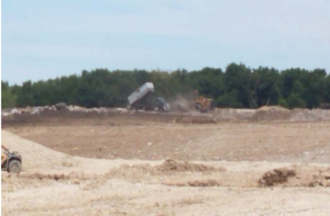
Tipping of truck in Northeast of Phase 1 of North Expansion West
