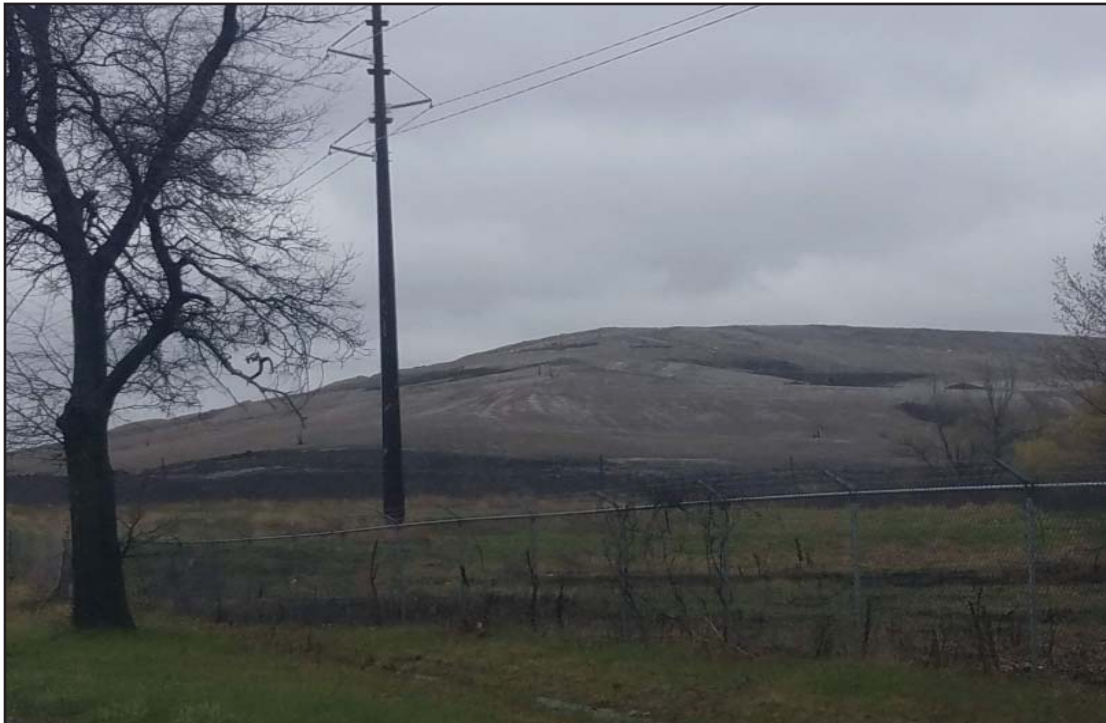
Cap development for Clearwater Pond Expansion
