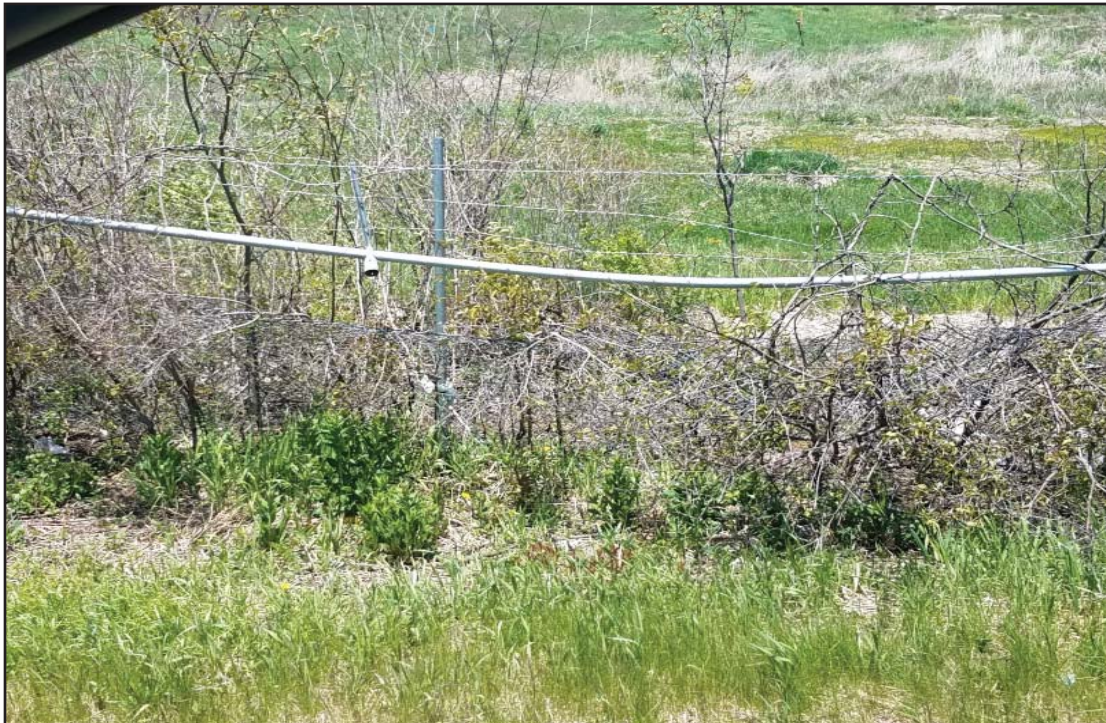
South section of perimeter fence in need of repair
