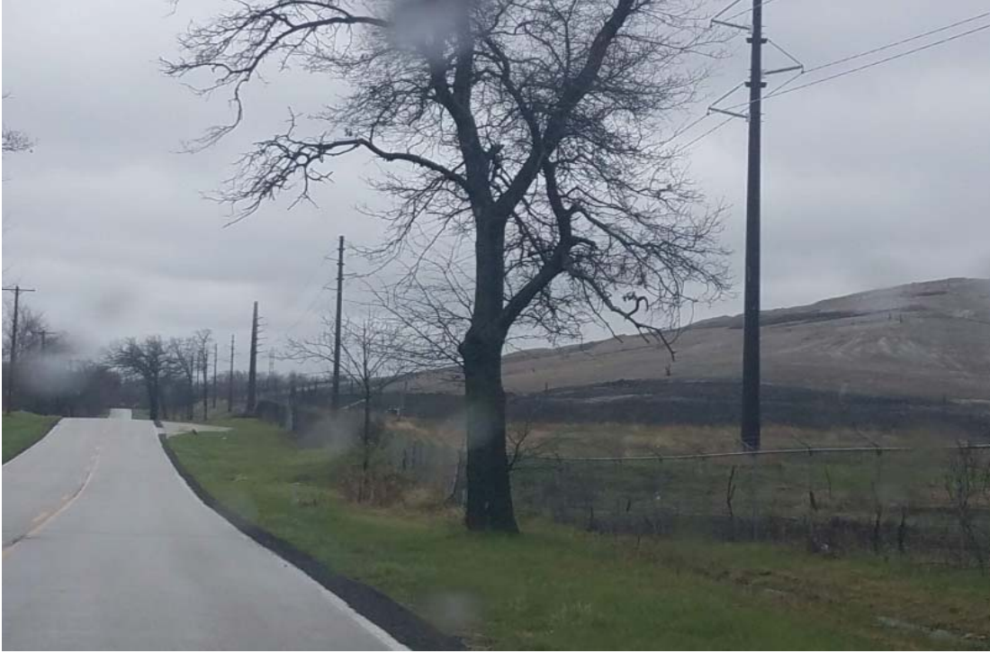
Cap development for Clearwater Pond Expansion
