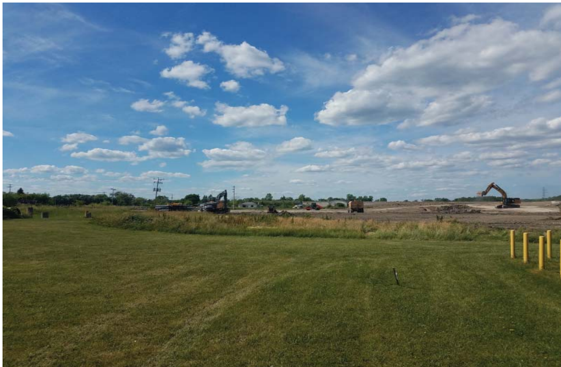
Excavation of new temp sed basin at North end of North Expansion West
