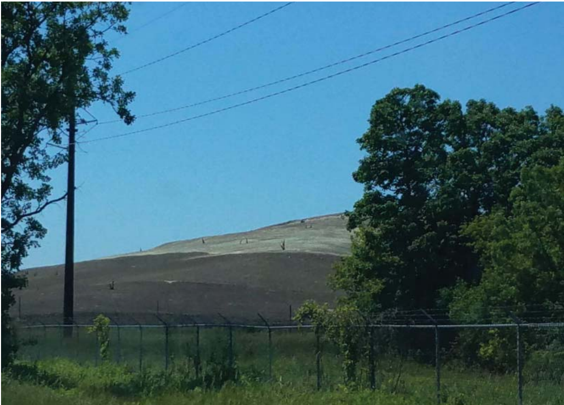
Cap development for Clearwater Pond Expansion
