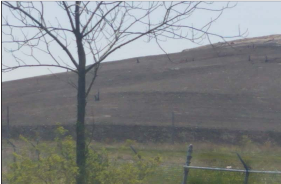
Cap development for Clearwater Pond Expansion
