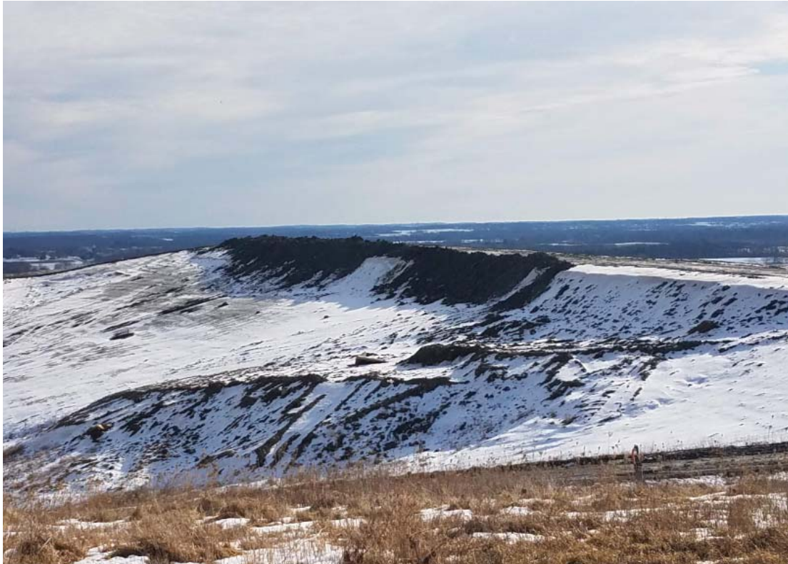
Soils being stockpiled on top of Phases 6 & 7
