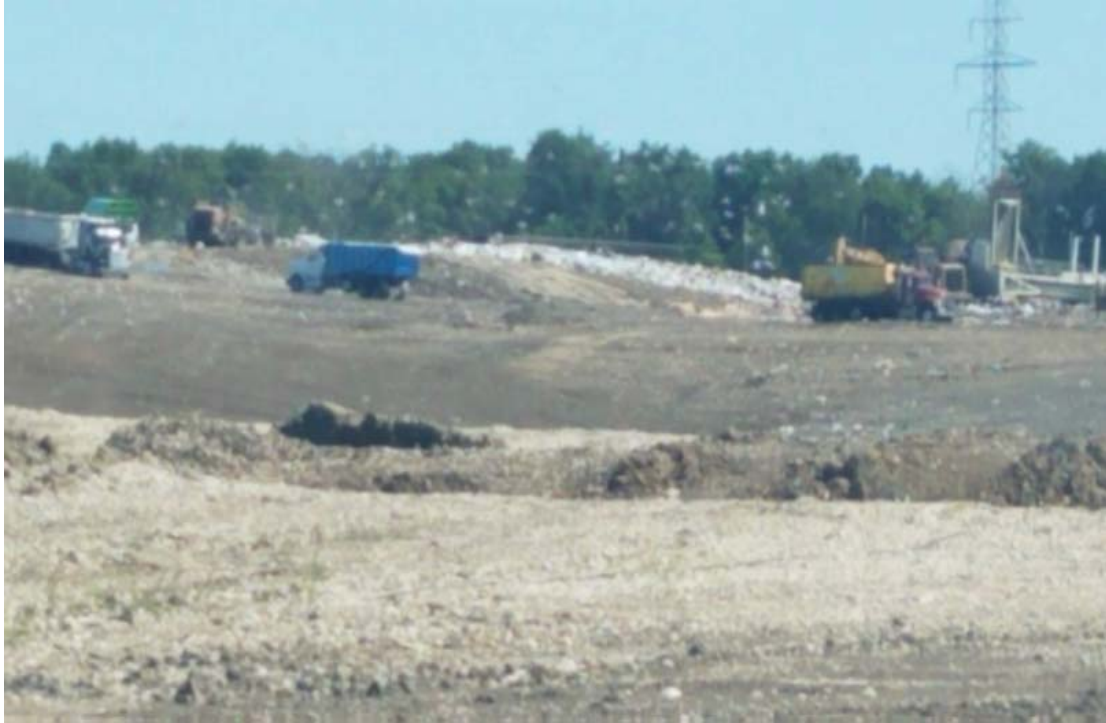
Waste being pushed North of Tipper
