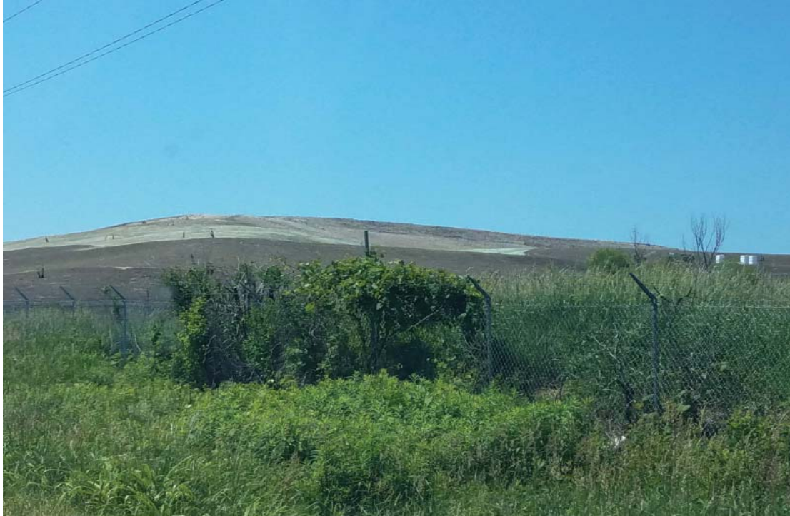
Cap development for Clearwater Pond Expansion
