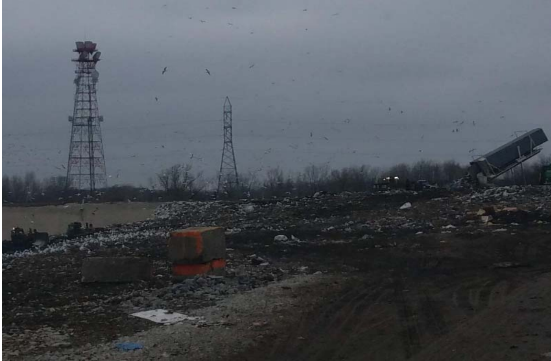
Overview of North Expansion West (NEW) viewed from the South
