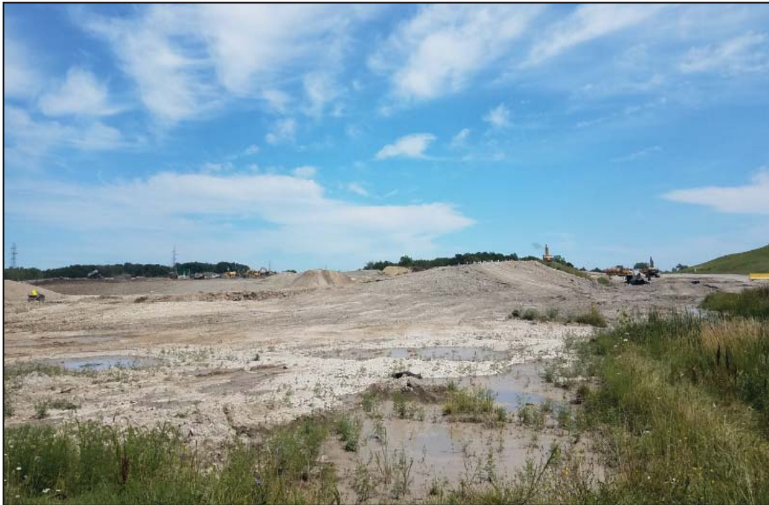
Completed berms and areas above Phase 2B of North Expansion west
