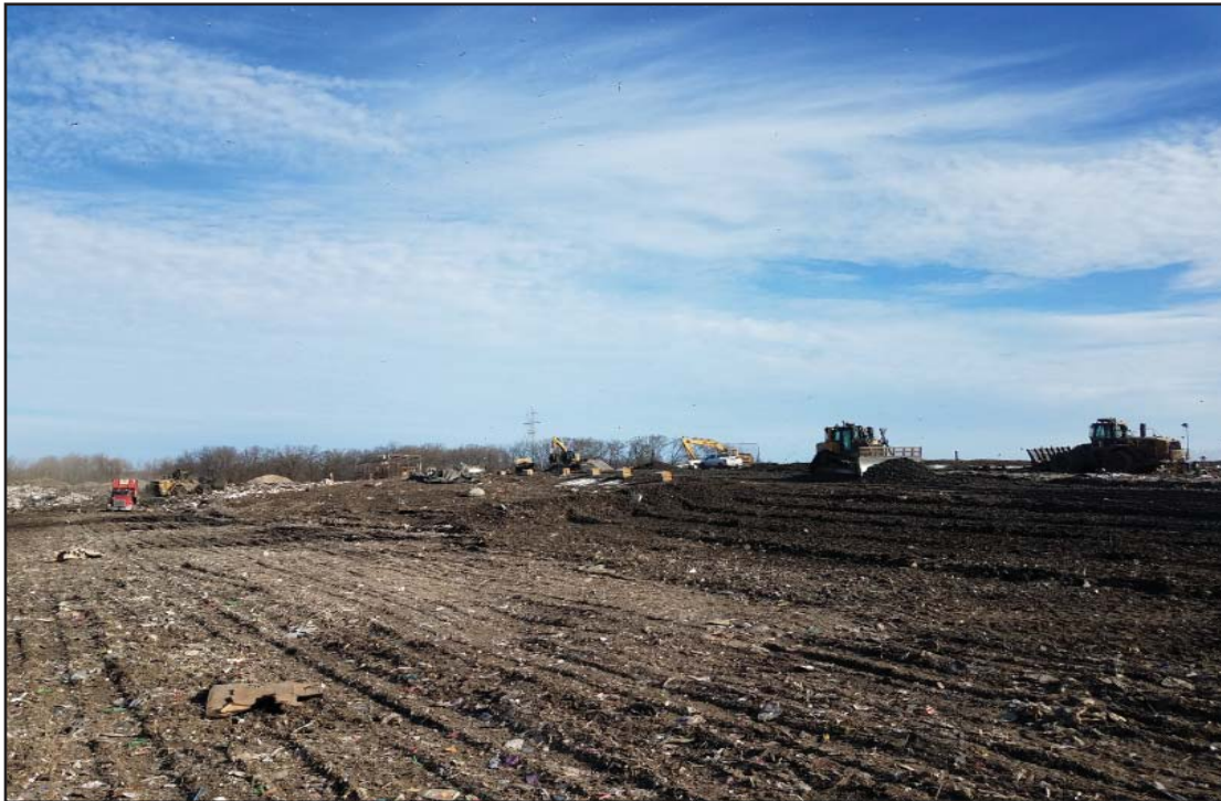
North Expansion West, looking North, new access road construction on the right
