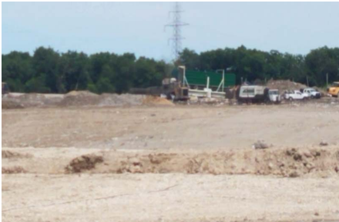
Tipper in middle of Phase 1 of North Expansion West
