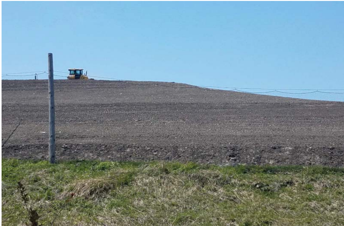
Cap development for Clearwater Pond Expansion
