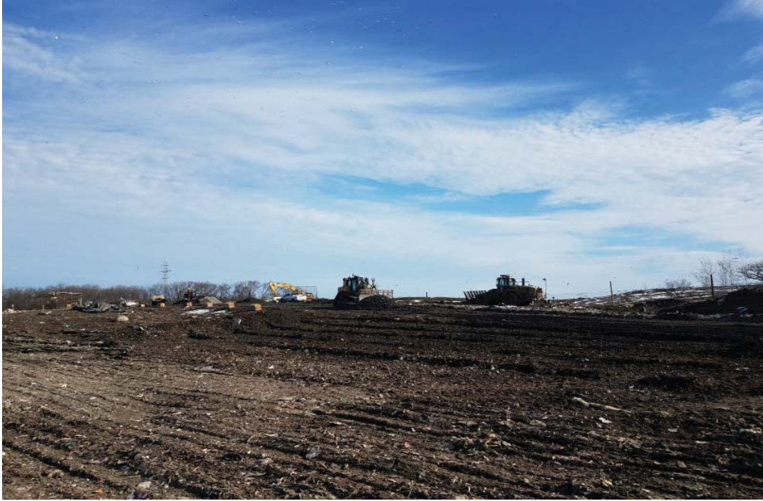
Spreading of stone to make a travelway for new access road in North Expansion West
