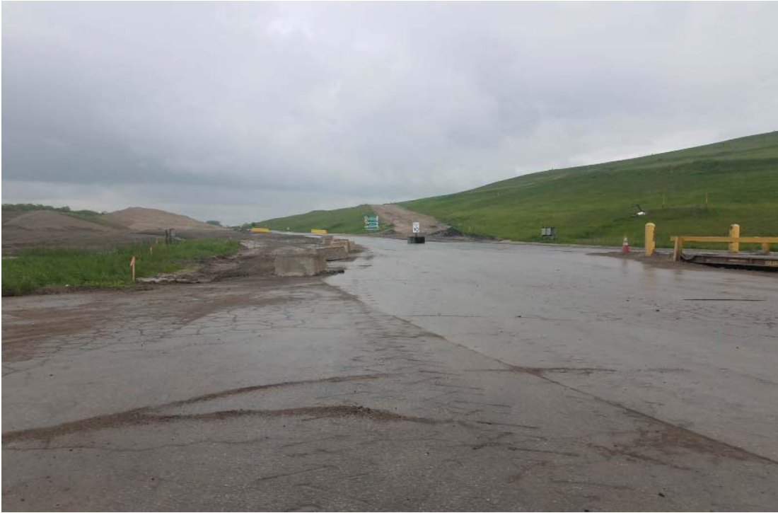
Newly paved, start of new paving going Eastward to North Expansion West (NEW) entrance
