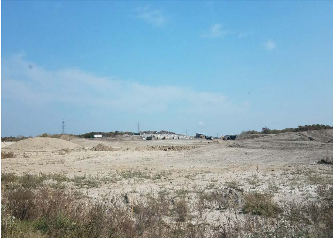
Overview of North Expansion West, viewed from the West
