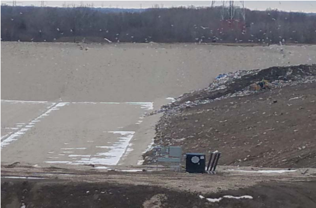
Dozer pushing waste down to Phase 2A of North Expansion West (NEW)
