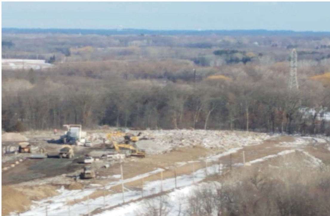
Working face at North end of North Expansion West
