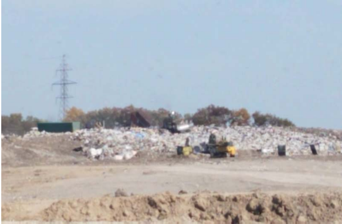
Working face in center of North Expansion West, lyft has crested out of excavation area
