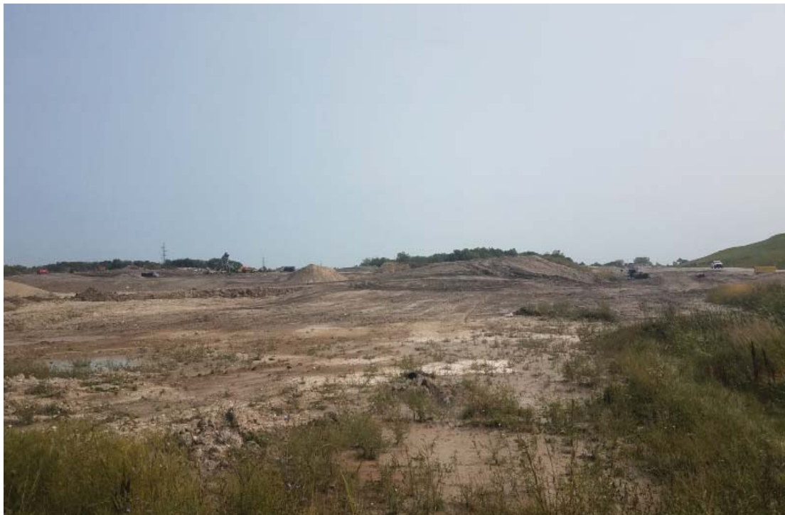
Phase 1 of North Expansion West, viewed from West
