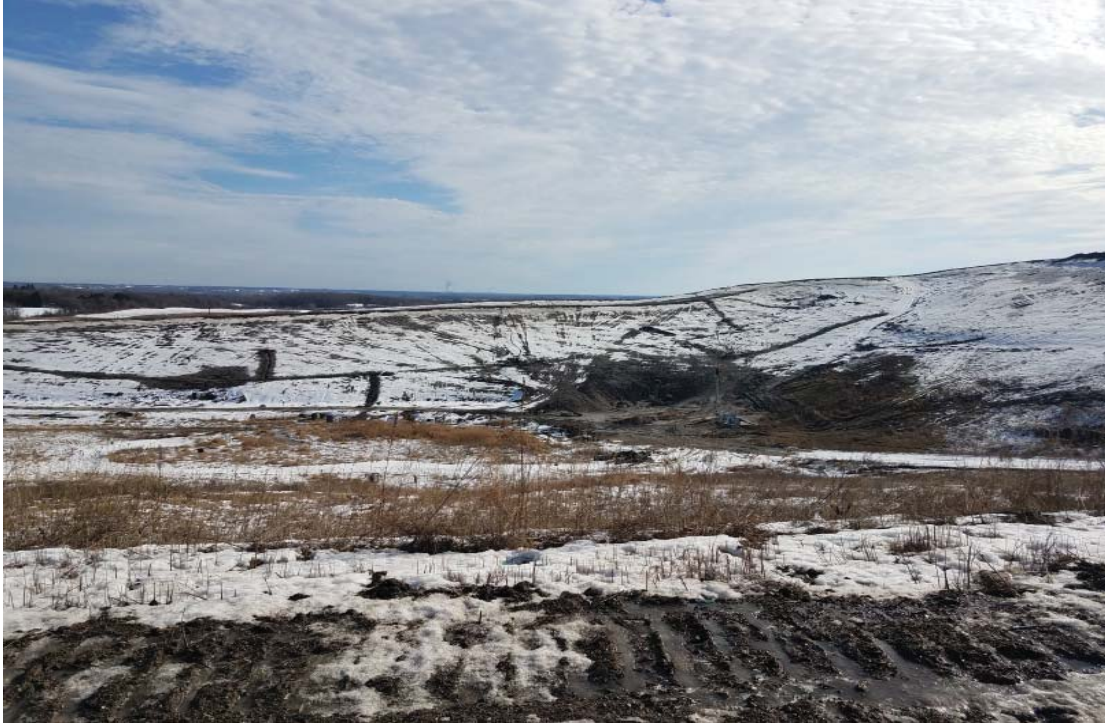
Clearwater Pond Expansion West slope, melted snow over gas headers
