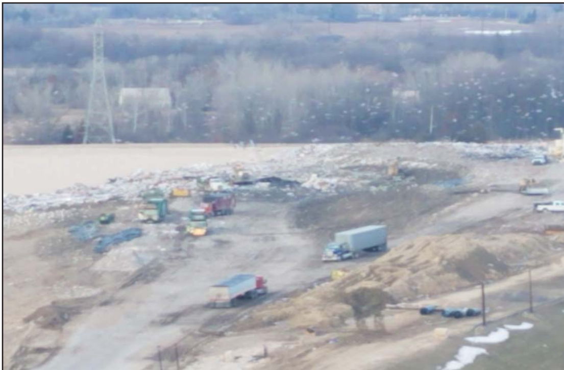
Active area of North Expansion West
