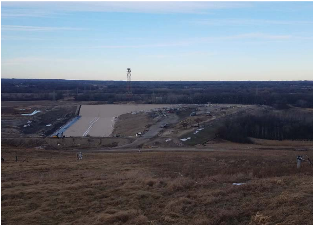
Photo from 01/06/2020, overview of North Expansion West (NEW) before waste placement
