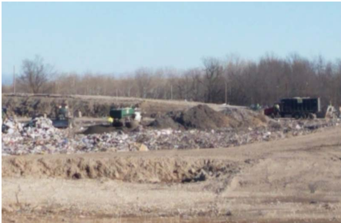
South end of Phase 2A, cover soils stockpiled at edge of active area
