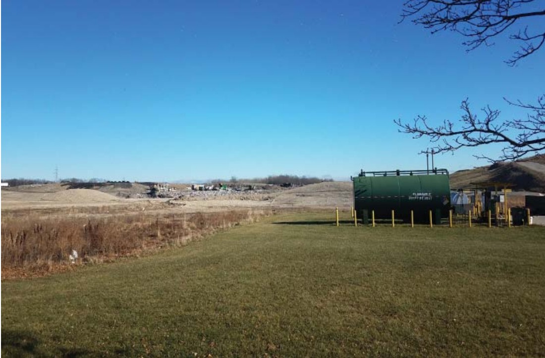
Overview of North Expansion West viewed from West
