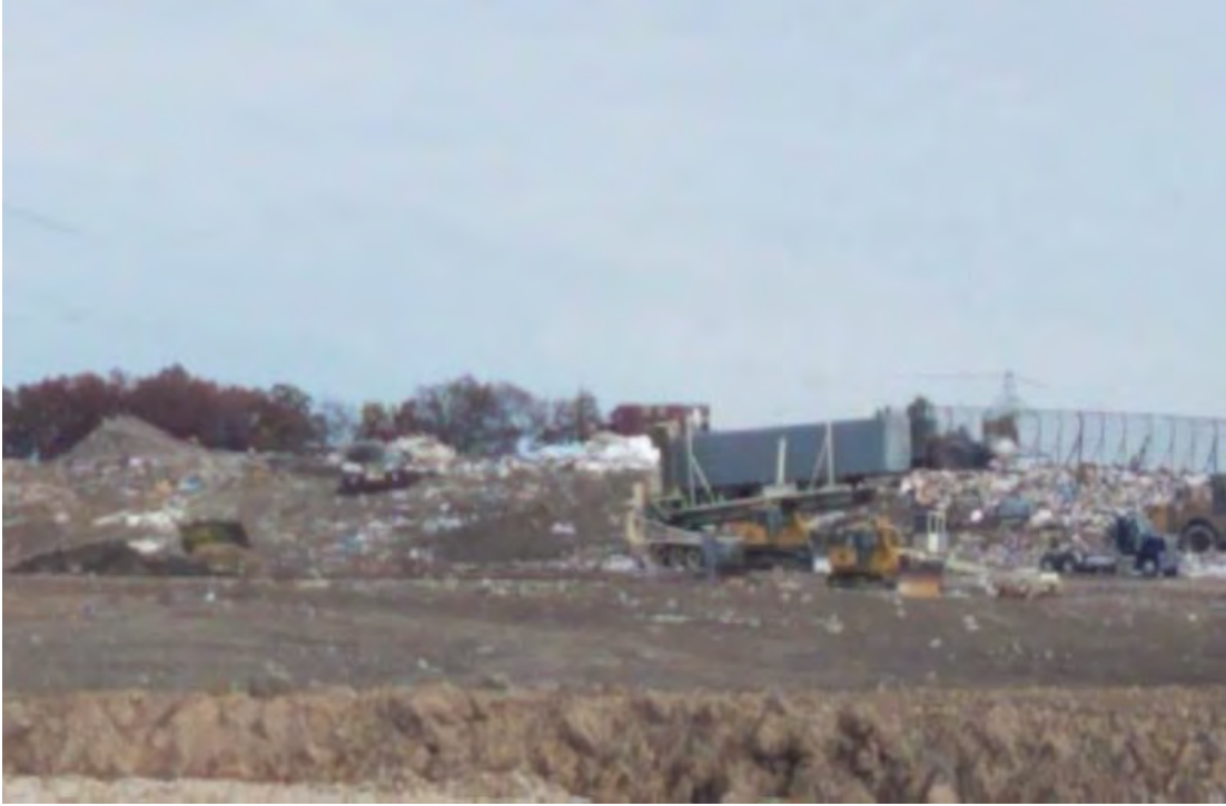
Northern end of Phase 1A of North Expansion West, receiving cover
