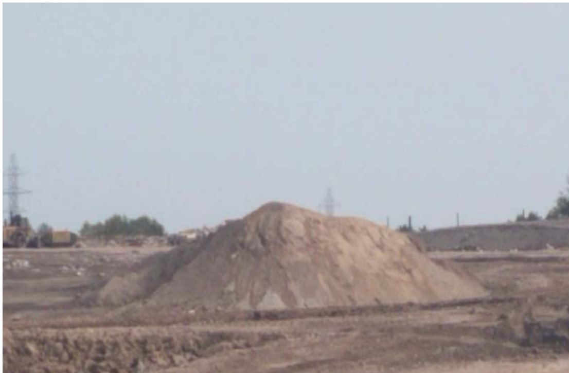
Boundary berm at South end of North Expansion West (NEW)
