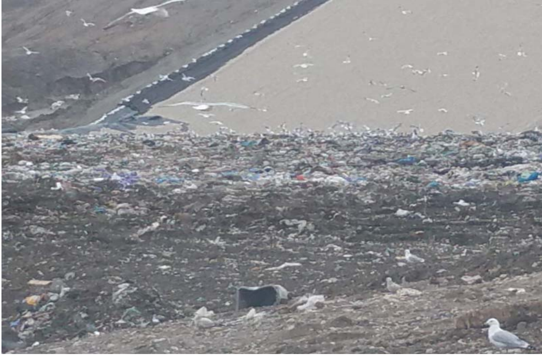
Layer of waste above fluff layer on Phase 2 of North Expansion West (NEW)
