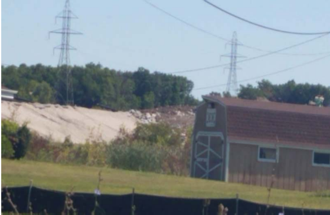
Exposed drainage blanket for Phase 2B of North Expansion West
