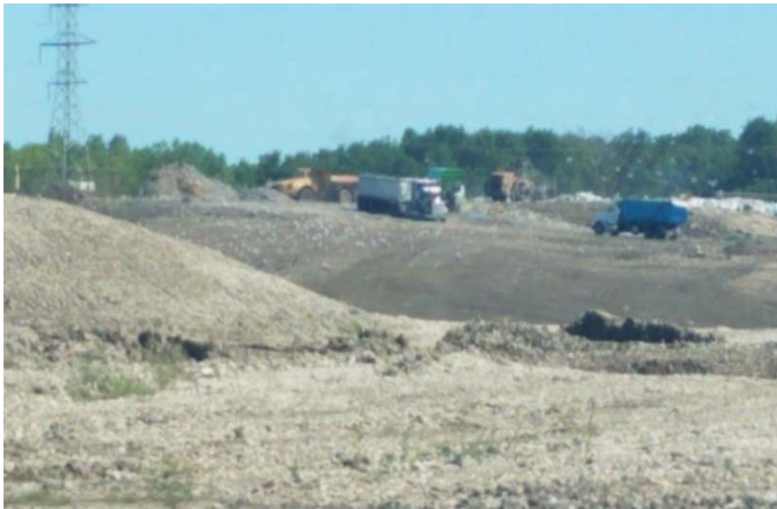
Trucks tipping at far end of Phase 1 of North Expansion West
