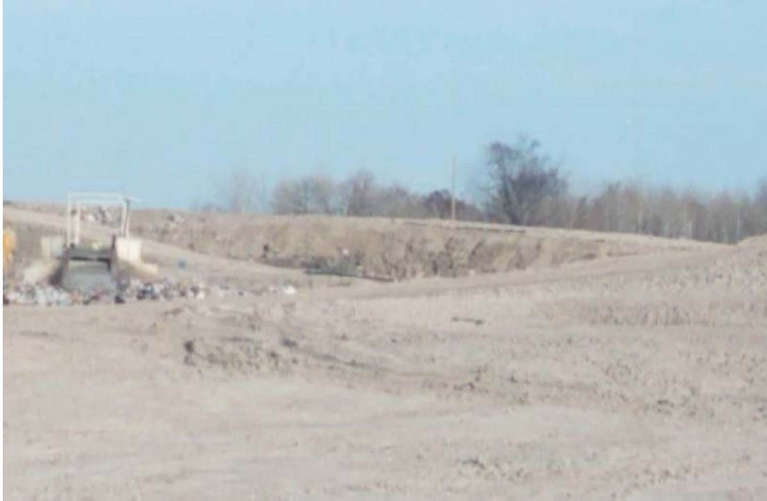
South end of Phase 2A, still below grade
