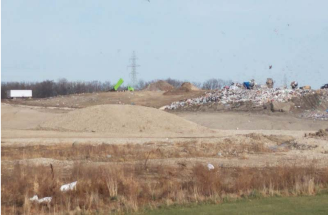
Working face and soil moving in Phase 1B
