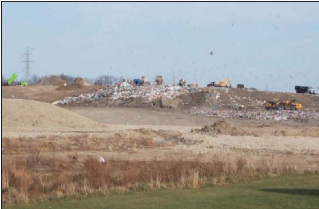
Upper elevation Working Face in Phase 1B
