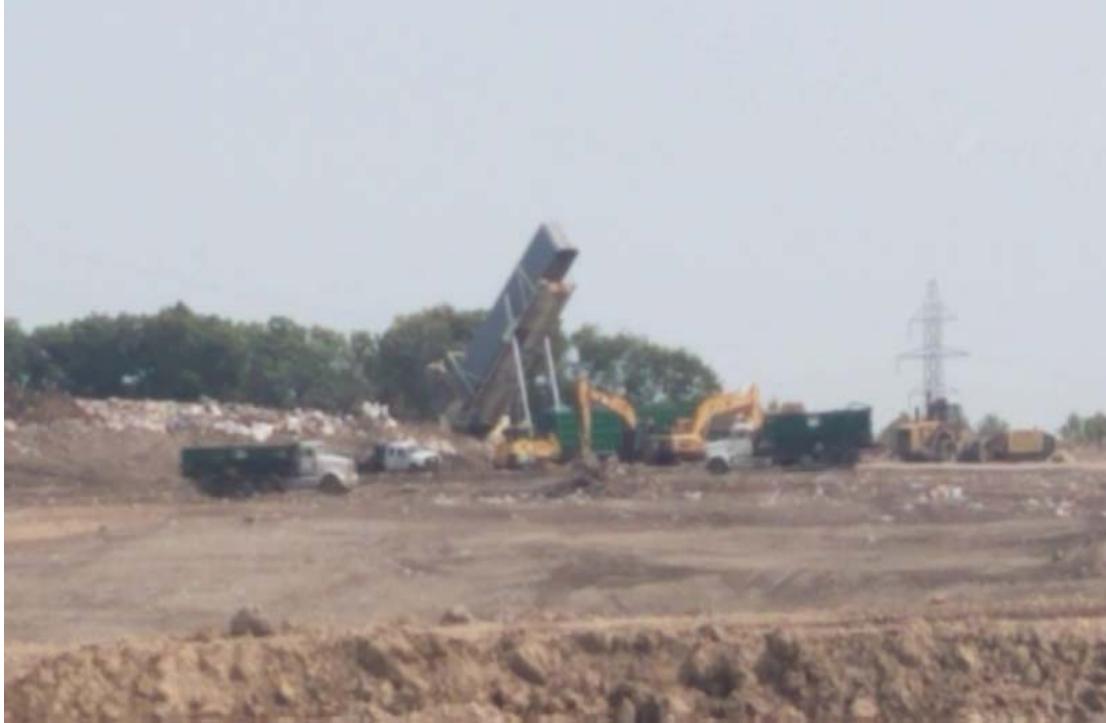
Waste being pushed North of Tipper
